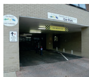
Poorly integrated car parking entrance
