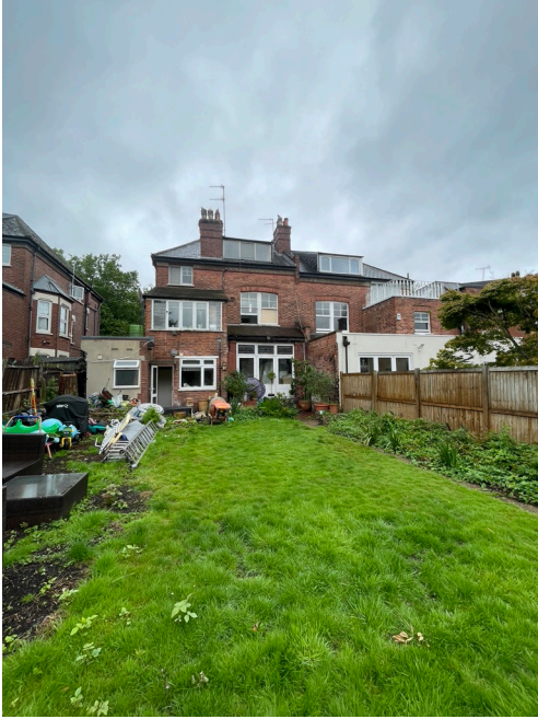
Rear Elevation Taken 5-08-23
