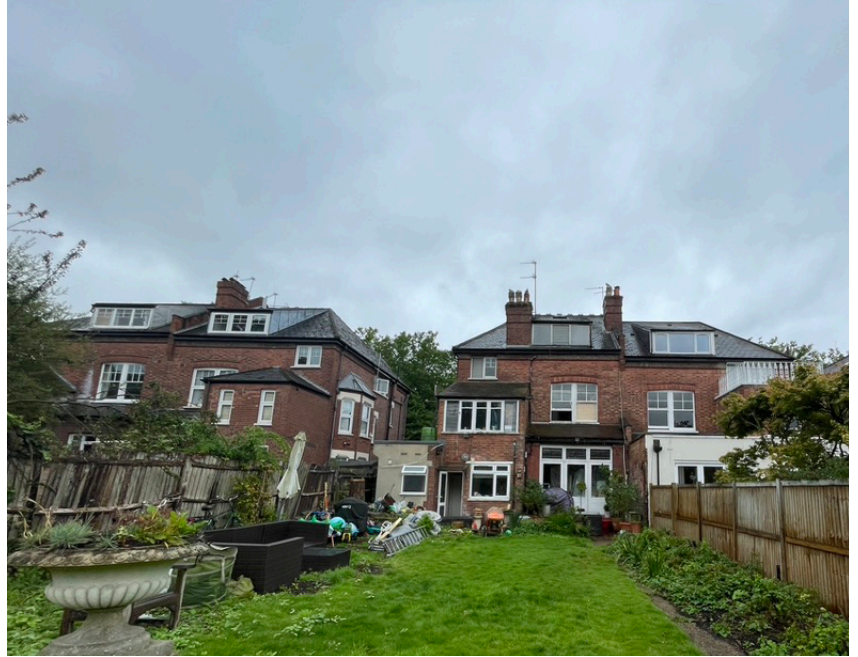
Rear Elevation Taken 5-08-23
