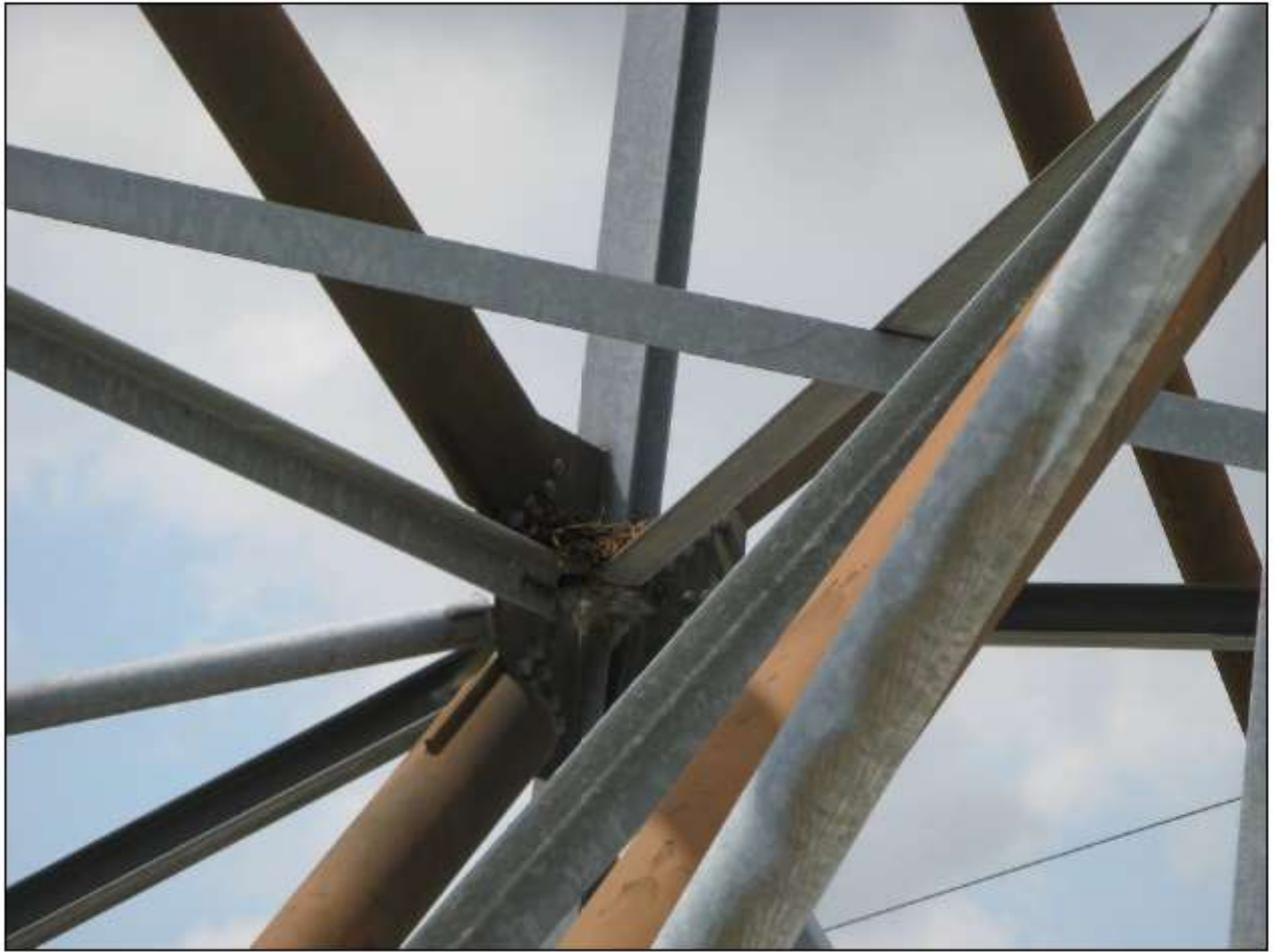
Photo L – more distant shot of same crow nest at girder junction
