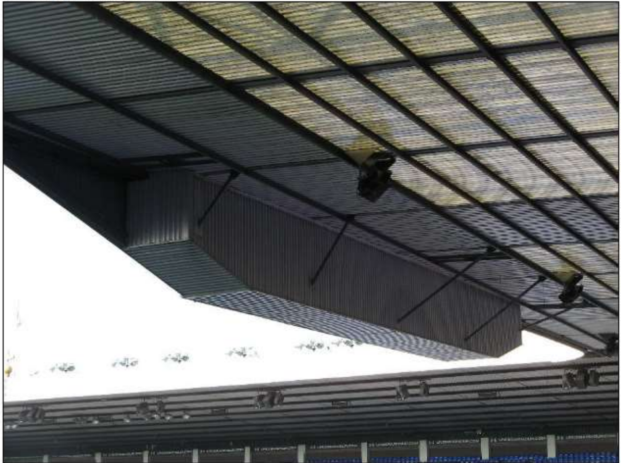
Photo B – more distant shot of the rear lower half of the north stand monitor that is used by the nesting kestrels
