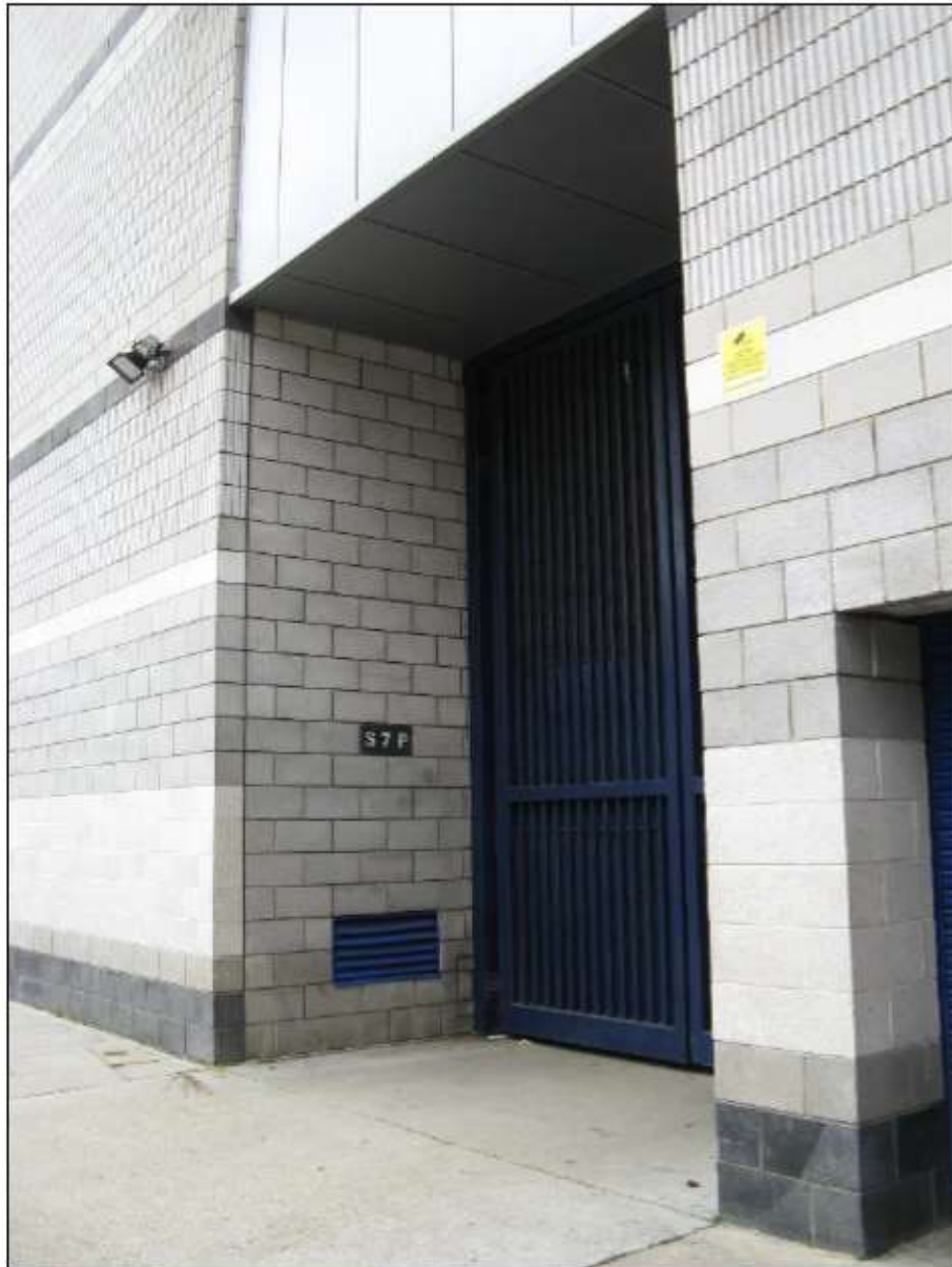
Photo J. The door and location directly below the overhang with the starling nest hole as shown in Photo I.
