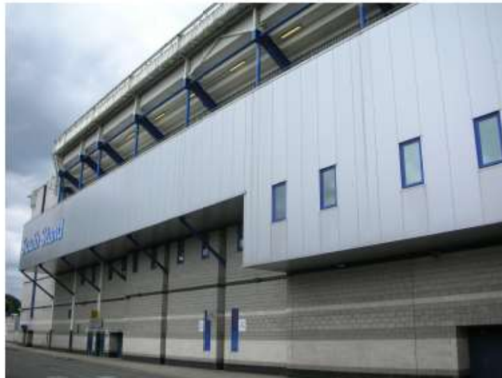
Plate 1 - Stadium, view from Park Lane facing west.
