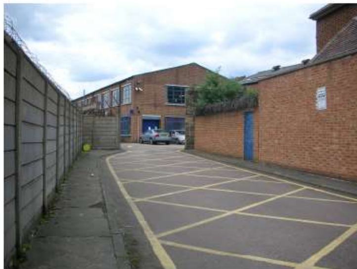
Plate 8 - Offices by the industrial estate, along Worcester Avenue facing west.
