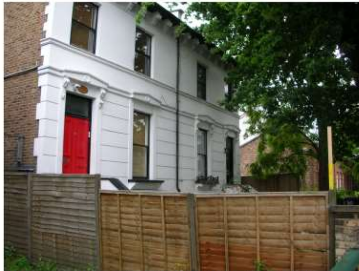
Plate 9 - Housing along Northumberland Park, facing south-west.
