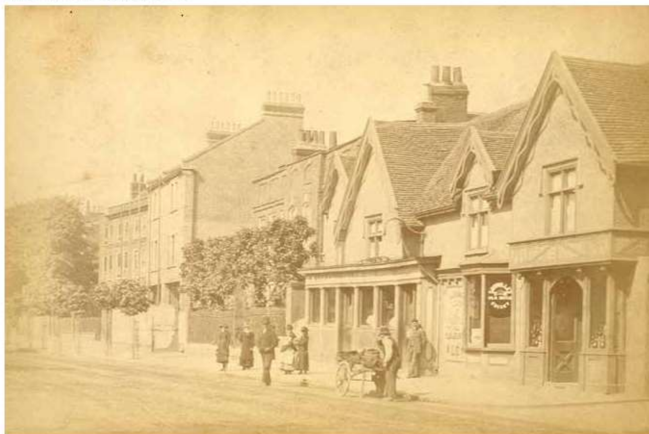
Figure 22. 750-755 High Road c1880-5
