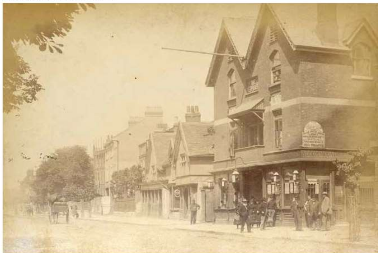
Figure 20. 748-756 High Road c1880-85
