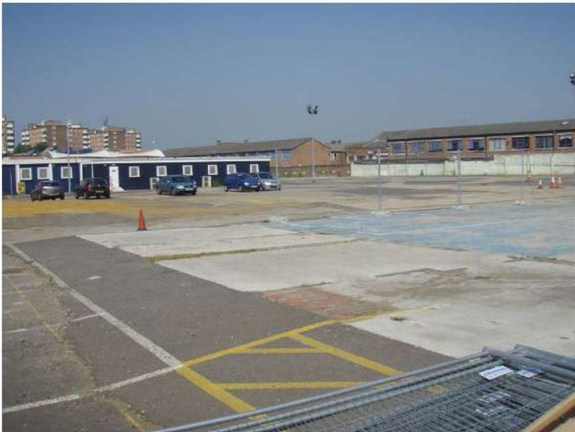
Photo 4: Looking northwest in the area of hardstanding immediately north of Paxton Road.
