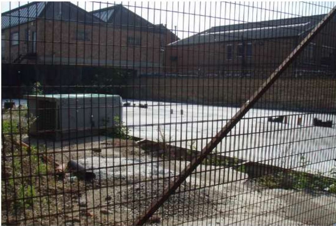
Photo 1 North of the Gibson Business Centre, looking south east at concrete slab and foundations.
