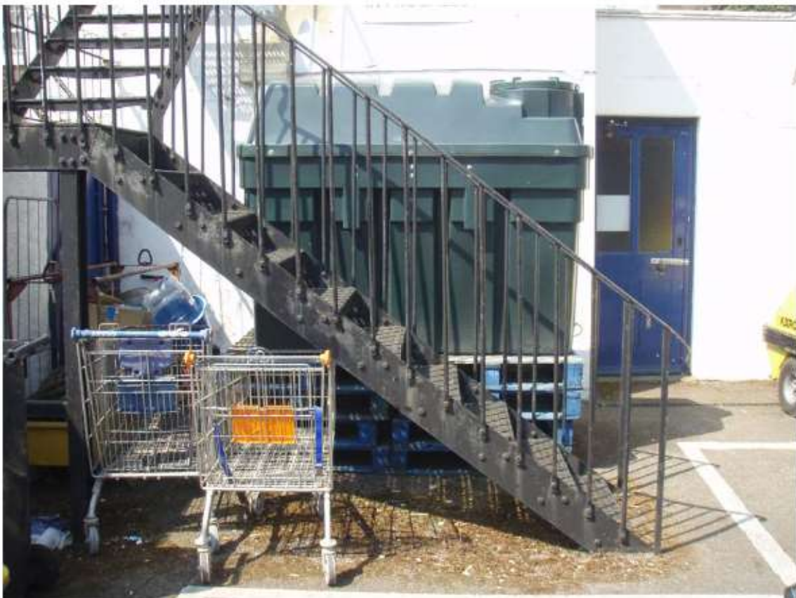
Photo 6 Looking west at diesel tank in Tottenham Hotspur Football Stadium main car park.
