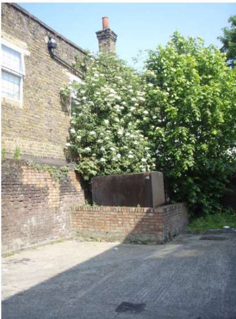
Photo 2 Looking north in Gibson Business Centre, a tank of unknown content.
