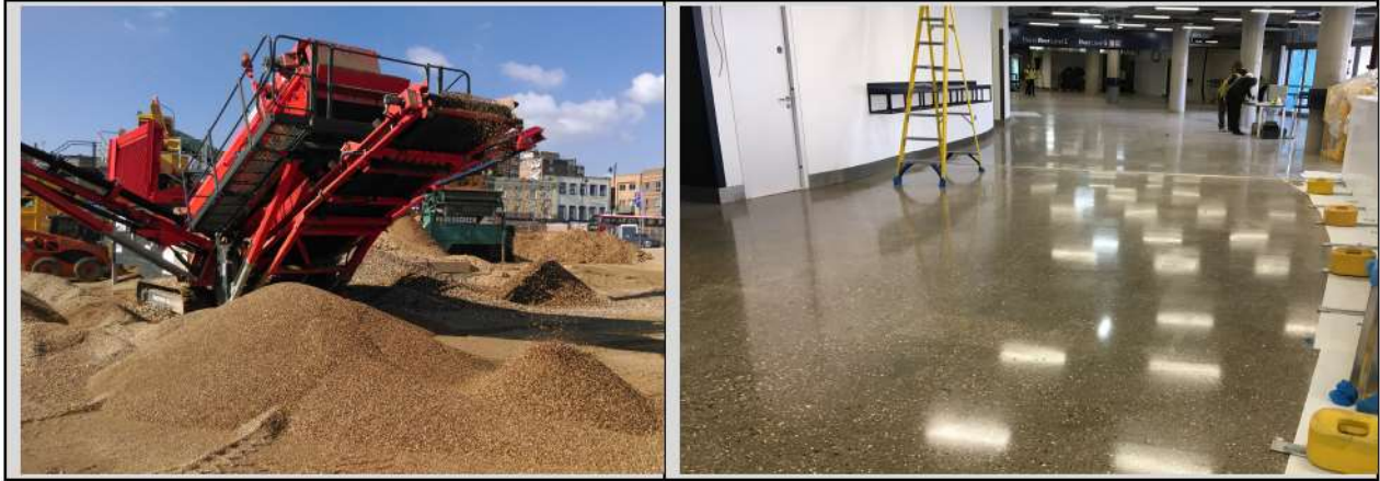
Figure 3-2 - Gravel washing plant and polished gravel slab using recovered excavated gravel from site at level one of the stadium west stand
