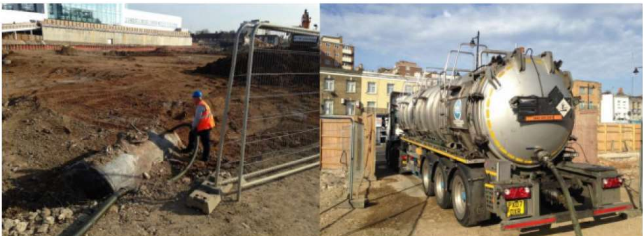
Figure 4.2 – Emptying of the UST on the 11/3/15 to tanker for disposal
