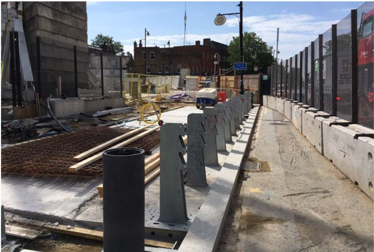
Figure 4-3 External hardstanding finishes being completed, block paving yet to be installed when this image was taken
