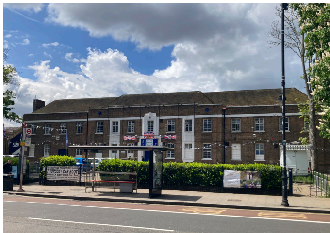
Fig. 6.24: The Tottenham Community Sports Centre at Nos.701-703 High Road.
