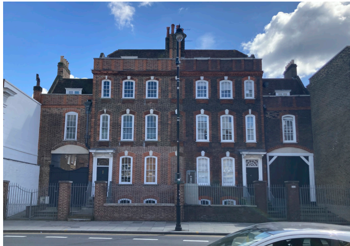
Fig. 6.16: Small scale terraced residential Grade II* premises at Nos. 808 and 810 High Road.
