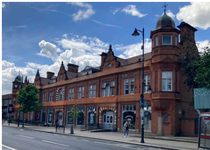
Fig. 6.20: The southern part of the North Tottenham Conservation Area as seen from the High Road near the junction with Lordship Lane. The Grade II listed No. 639 in the foreground.
