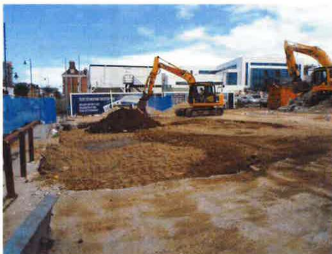
Plate 3: Extent of the excavation following the removal of the underground tanks.
