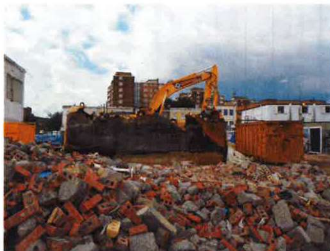
Plate 4: One of the tanks awaiting cutting up and removal from site.
