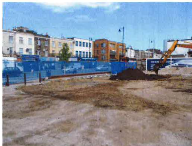
Plate 2: Site of the former tank farm at the front of the site, adjacent to the road.
