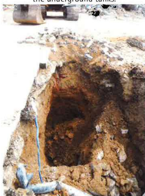
Plate 5: Trial pit (V1) in the north of the former tank farm area.
