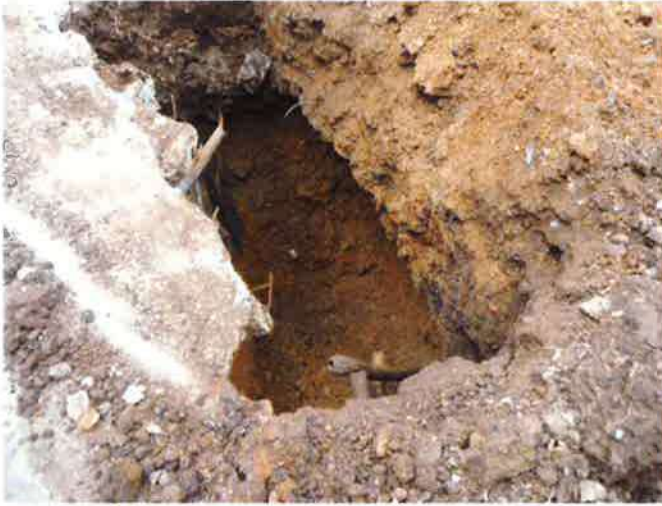
Plate 7: Trial pit (V2) in the east of the former tank farm area.
