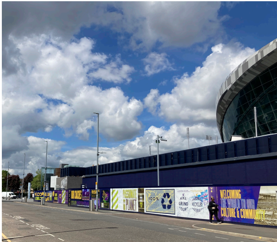
Fig. 3.8: Park Lane looking north-west with the unbuilt Plots 5, 4 and 3 and the completed Tottenham Experience buildings at Plot 2. The Stadium (Plot 1) is seen to the right.
