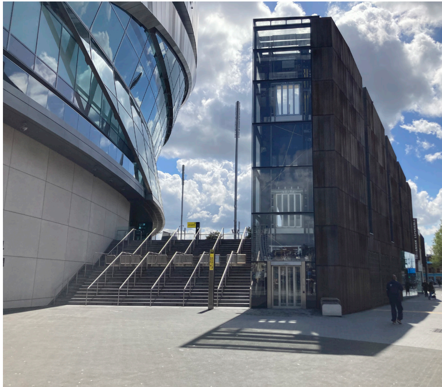
Fig. 3.5: The Stadium (Plot 1) to the left and the Tottenham Experience buildings on the High Road (Plot 2) to the right have been completed and are operational.
