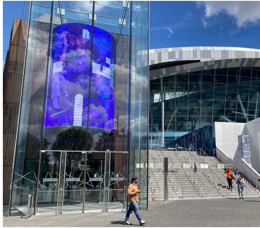
Fig. 3.6: The Tottenham Experience buildings on the High Road (Plot 2) to the left and Plot 3 to the right. The Stadium (Plot 1) is seen in the background.
