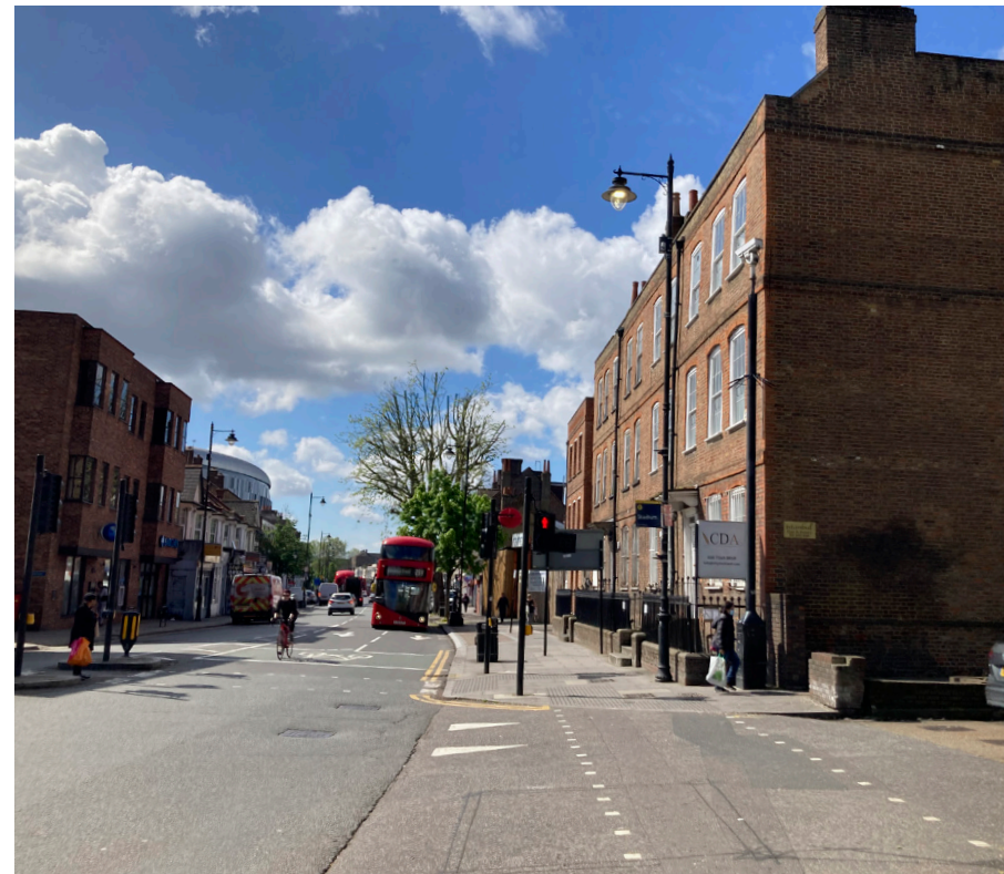
Fig. 3.12: View of the High Road and part of the North Tottenham Conservation Area. The Grade II listed Nos. 867 and 869 are in the foreground.
