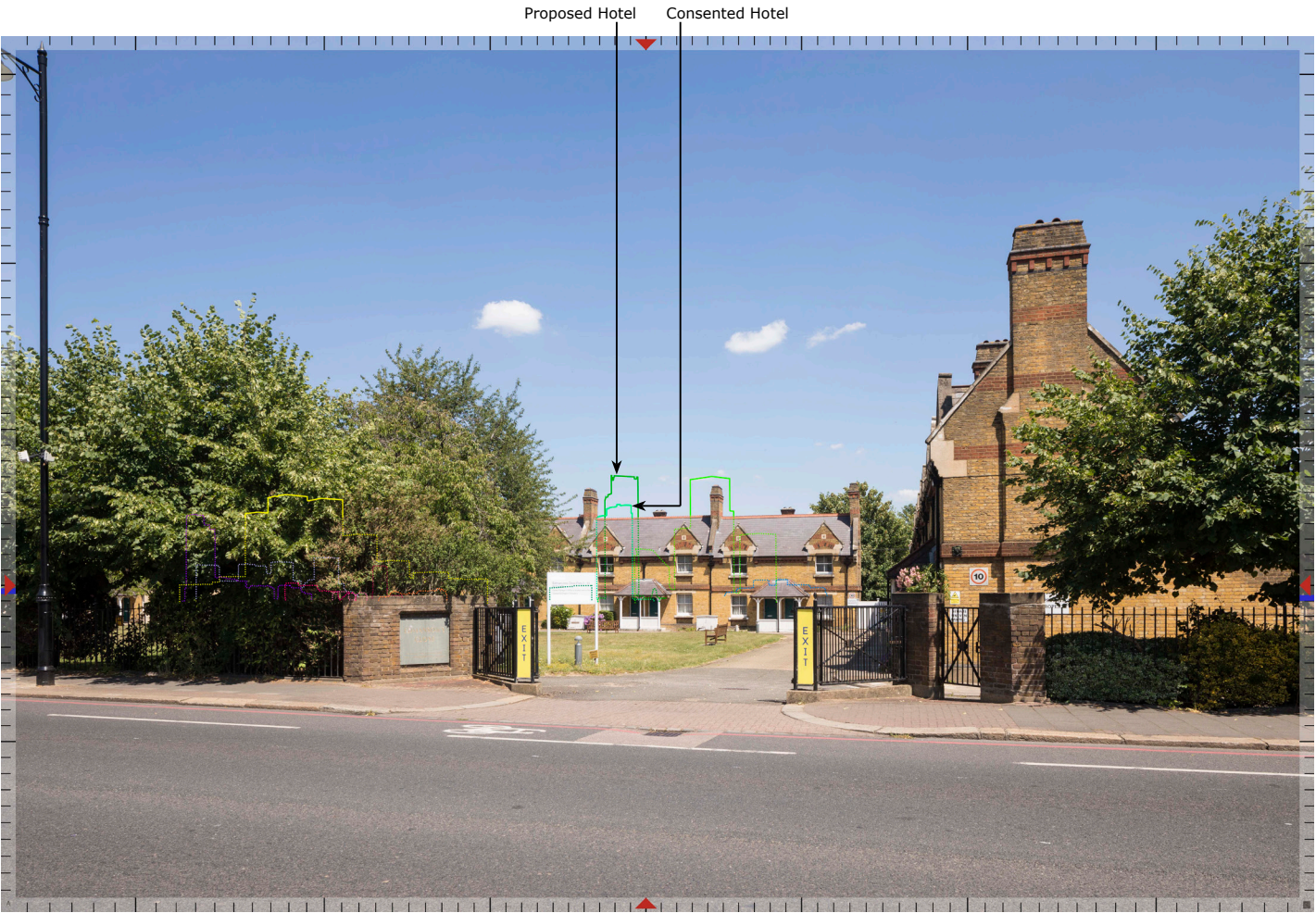
VIEW 14 - BRUCE GROVE LOOKING TOWARDS EDMANSONS CLOSE
