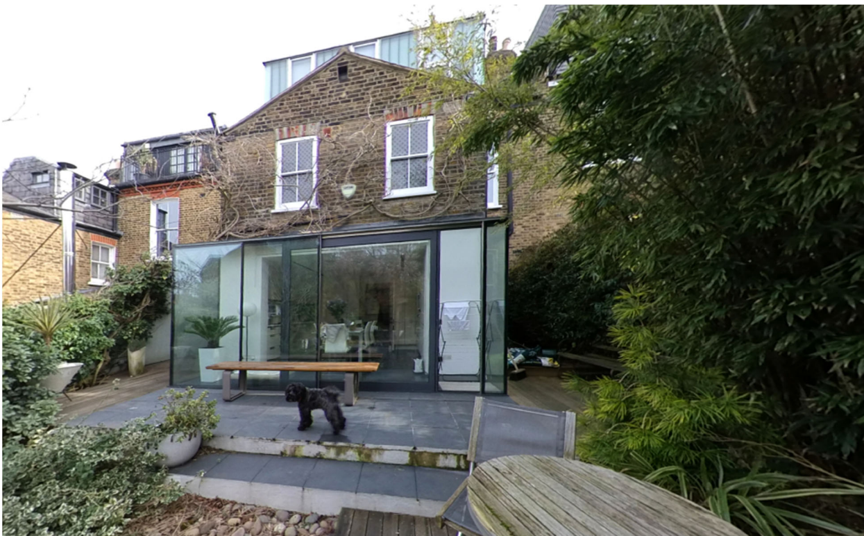
Fig. 04 Existing view of the rear of 19 Womersley Road
