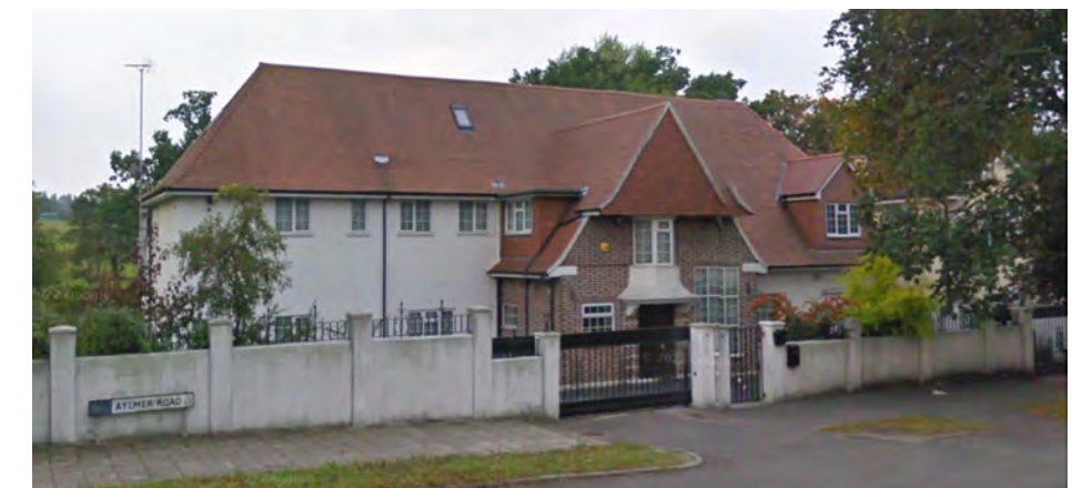
2. View of the front elevation of 27 Aylmer Road in September 2009 before the partial demolition of the east wing consented under planning permission ref. HGY/2009/1002
