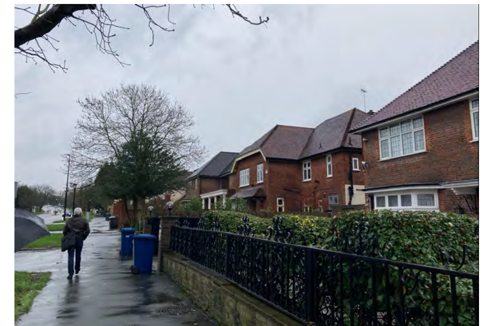
View along Aylmer Road looking east showing no.1 on the right in the foreground with no.3 in the middle and no.5 beyond to the left.
