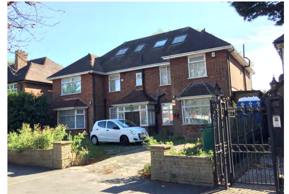
19 Aylmer Road mirrors the form of no.21 but has a different character given by the different porch and much plainer fenestration. Haringey Council granted consent for the house to be altered by the addition of single-storey side extensions on both sides and the conversion of the loft including removing the chimney and inserting roof lights in the front face of the roof under planning permission HGY/2016/2973.
