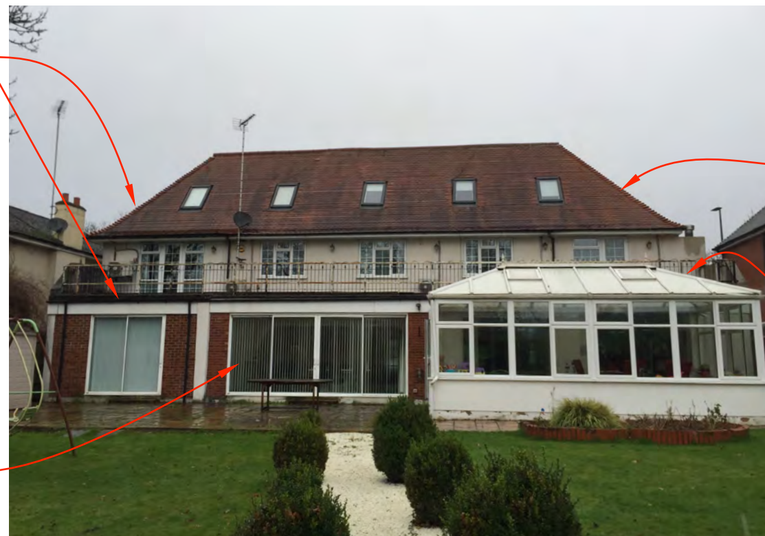
2. Rear Elevation viewed from the rear garden
