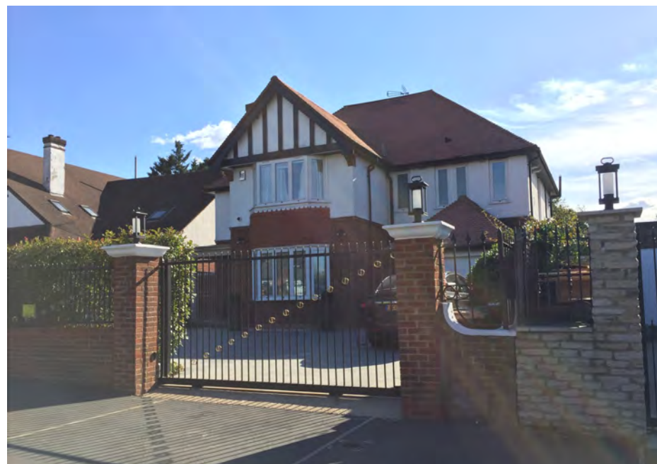
9 Aylmer Road and no.13 appear to have been built to the same original form and design, although each has subsequently been altered in different ways. The main volume of the house has a hipped roof and the two-storey projecting bay on the front elevation has mock-Tudor half-timbering. A single-storey extension has been added at the front to enlarge the integrated garage.
