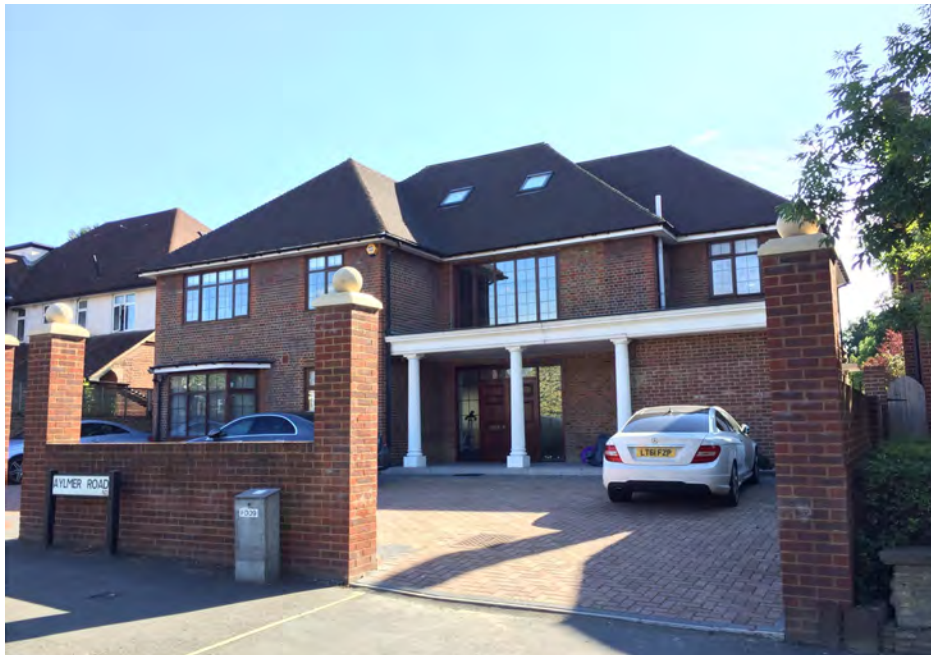
5 Aylmer Road was likely built to match No. 1 Aylmer Road, and has undergone some alterations since. The new alterations feature a classical-style porch with columns and entablature.
