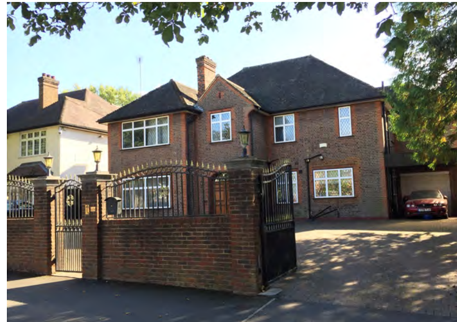
15 Aylmer Road has attractive red brick detailing at the external corners and around the window openings. Similar to the other houses along the row to the east the main volume of the house and the projecting bay at the front have hipped roofs but to create a central focus the two-storey bay at the position of the front door has a gable.
