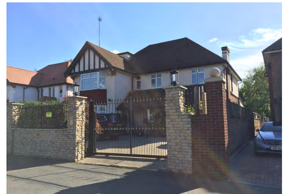
7 Aylmer Road is very similar in appearance to no.9 and no.13, the main difference being that the two-storey gabled projecting bay on the front elevation, rather than being set just off centre, is set to the left hand side. Haringey Council granted consent for the new porch that extends across the front elevation to be added under planning permission ref. OLD/1989/0084.
