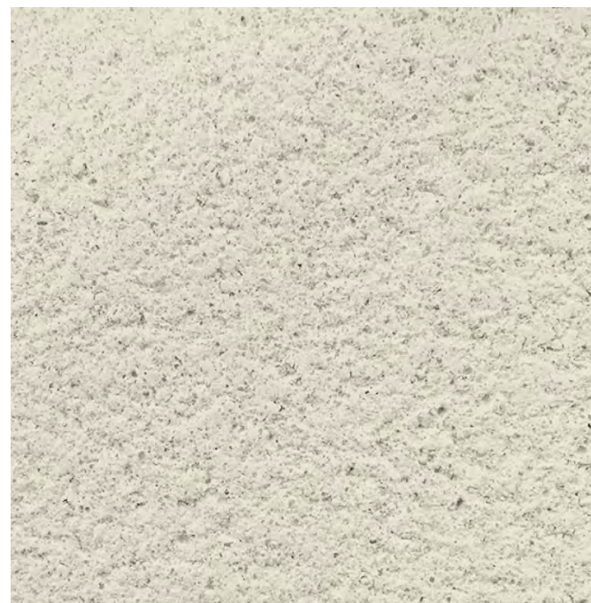
4. Pigmented, or painted render to the external wall at basement level
