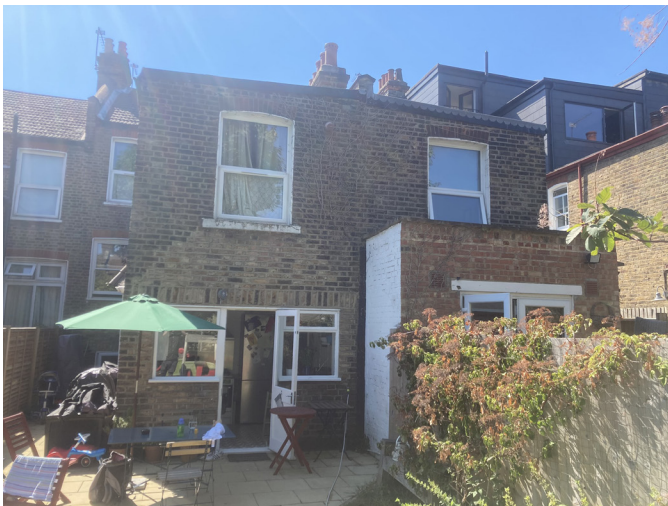
Rear view of kitchen windows and doors
