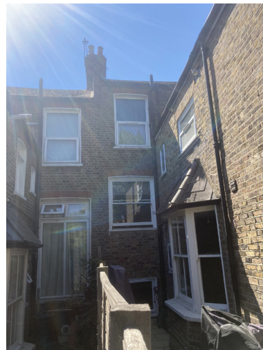
View of existing side bay windows
