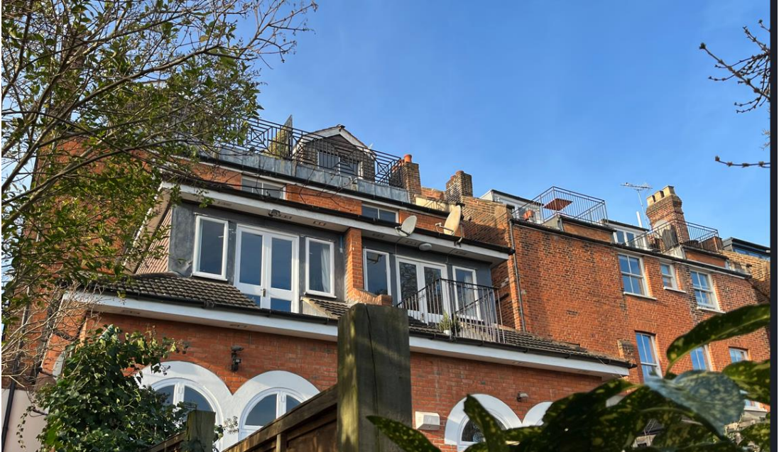
Existing balconies and windows that result in a degree of mutual overlooking at the application site
