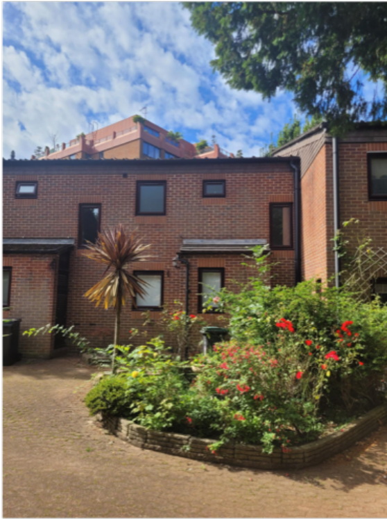
Front elevation of 6 Colwick Close
