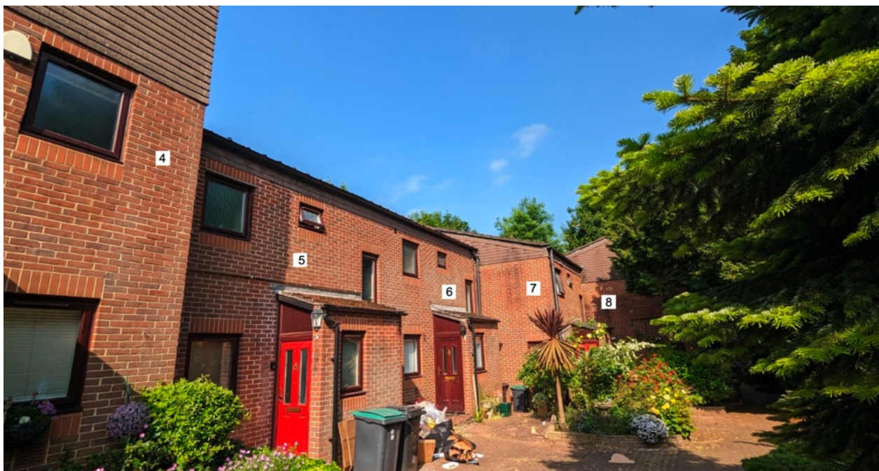
Street view of 4-8 Colwick Close
