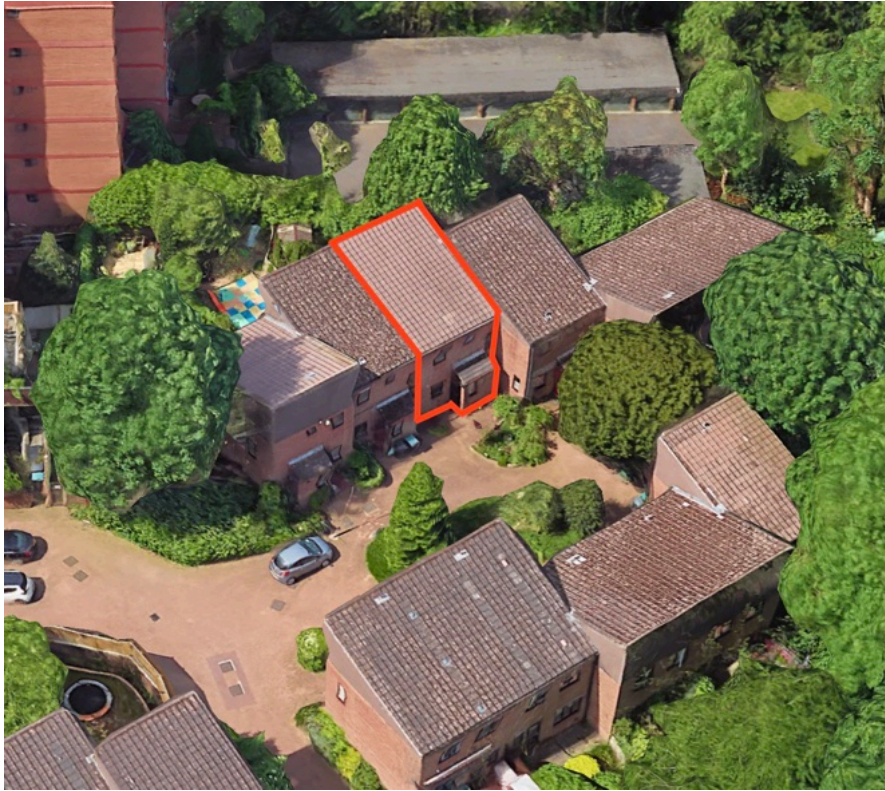
Aerial view from the front – property outlined in red.
