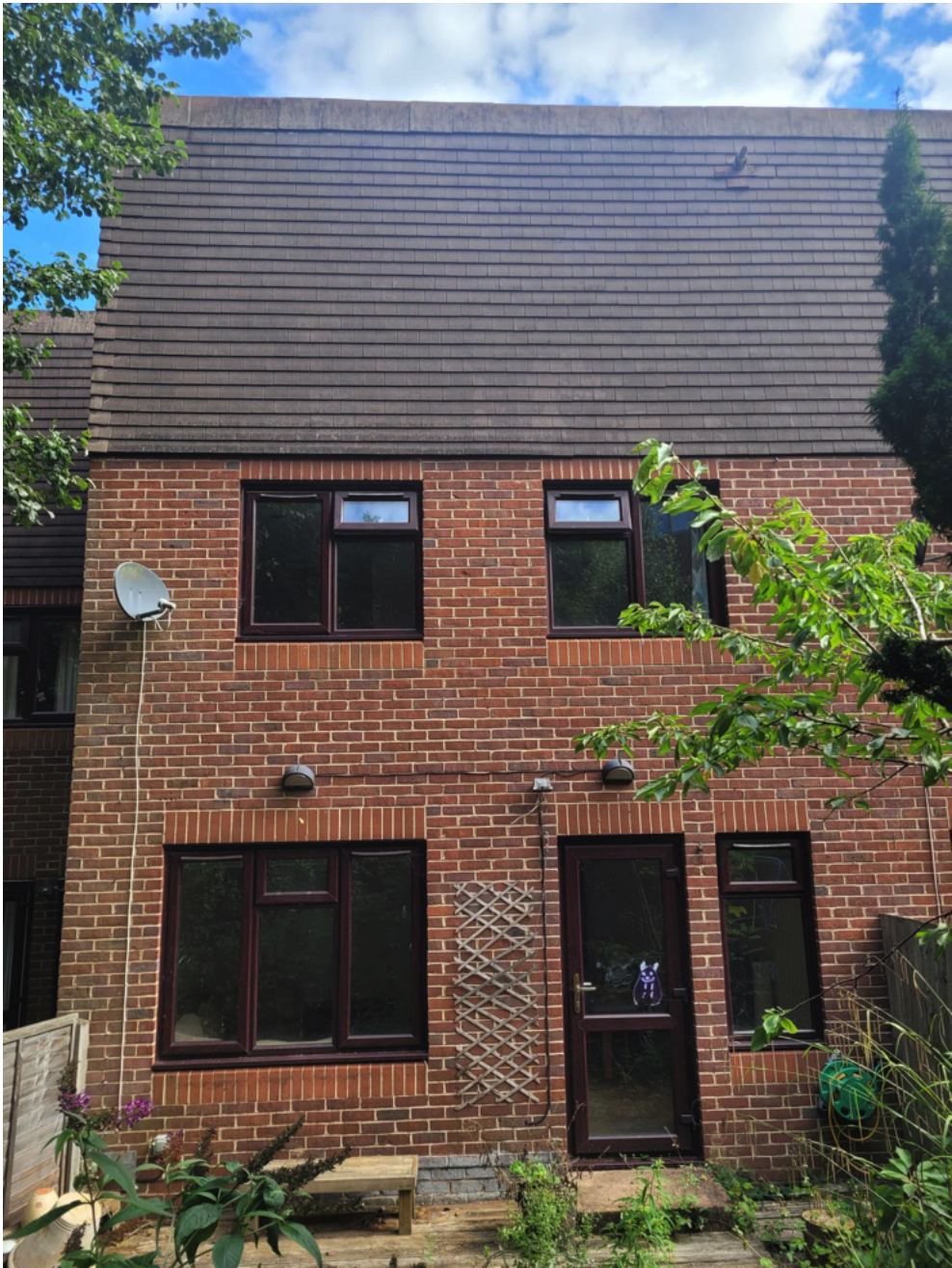
REAR ELEVATION, 6 COLWICK CLOSE (as seen from rear garden)
