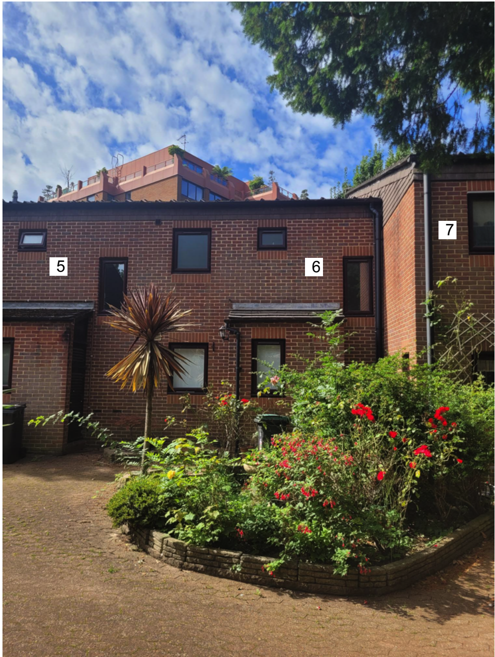
FRONT ELEVATION, 6 COLWICK CLOSE (as seen facing away from 11 Colwick Close)
