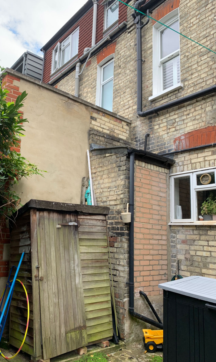
Concrete wall showing extension of property 57
