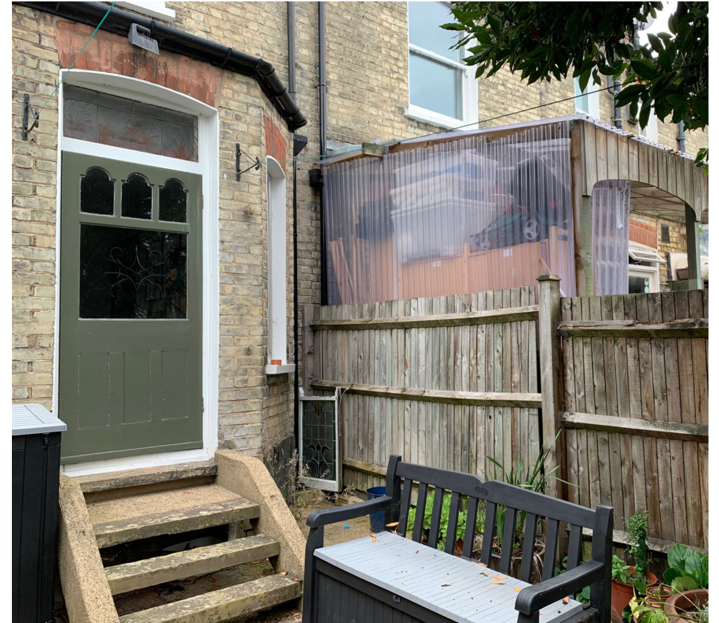
Fence / veranda cover of 61 property
