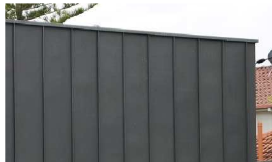
standing seam rainscreen cladding
