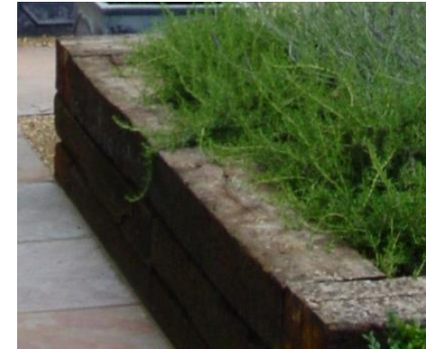
Fig13: raised beds for soft landscaping
