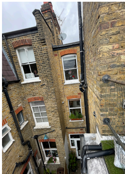
View from the second floor room (left) showing small side mansard and brick wall to be demolished and replaced with slate covered wall to match existing.
