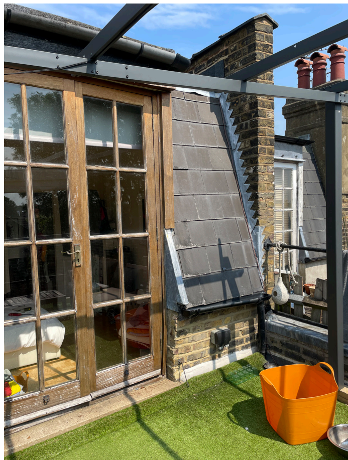
Existing rear mansard and roof terrace, looking towards no. 22 Alexandra Park Road.
