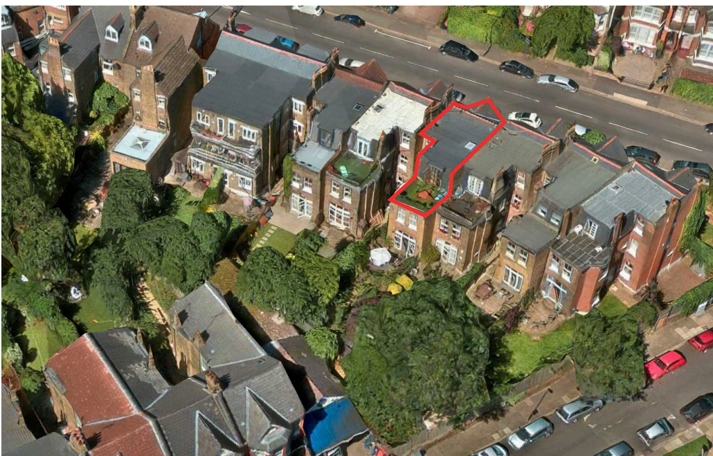
Aerial view highlighting terrace and roof of no. 20 Alexandra Park Road. The photo was taken prior to the extensions at no. 26 being built.
