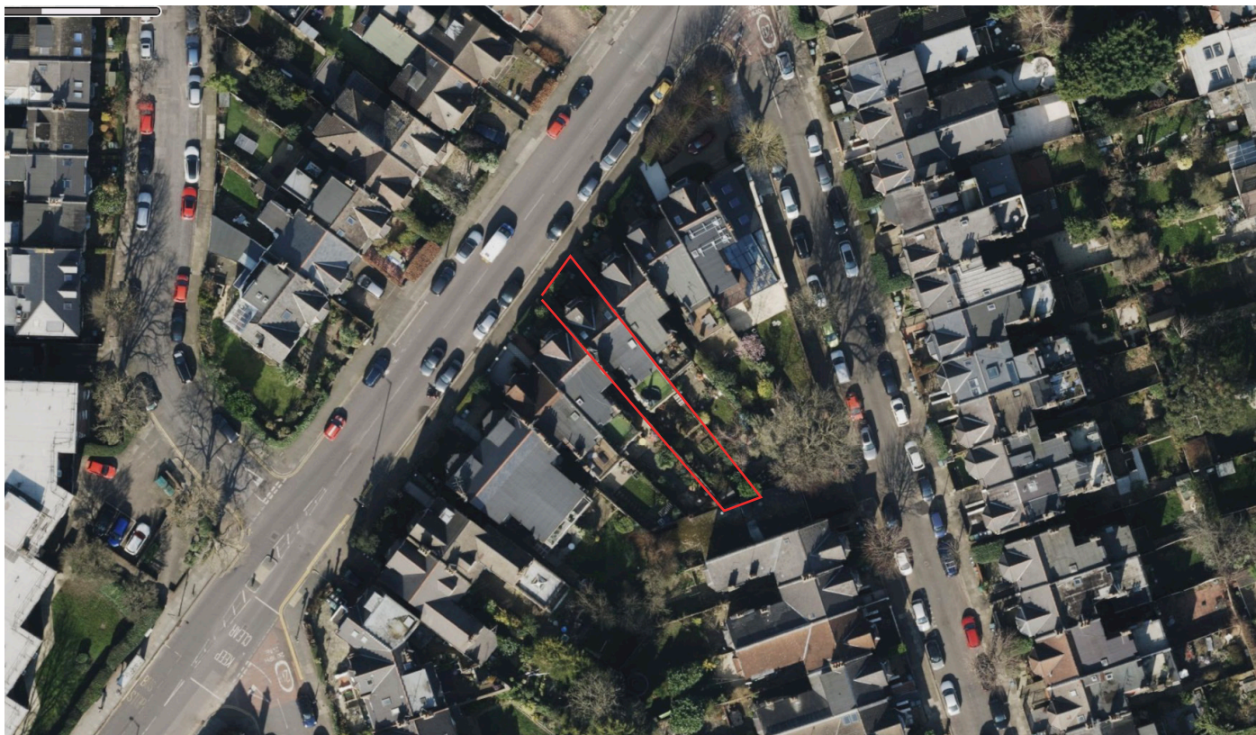
Aerial photo highlighting location of 20 Alexandra Park Road.
