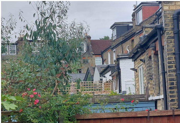
Fig. 6 Existing Rear view to left along the terrace, towards No.16, showing typical two pitched extensions between raised party walls
