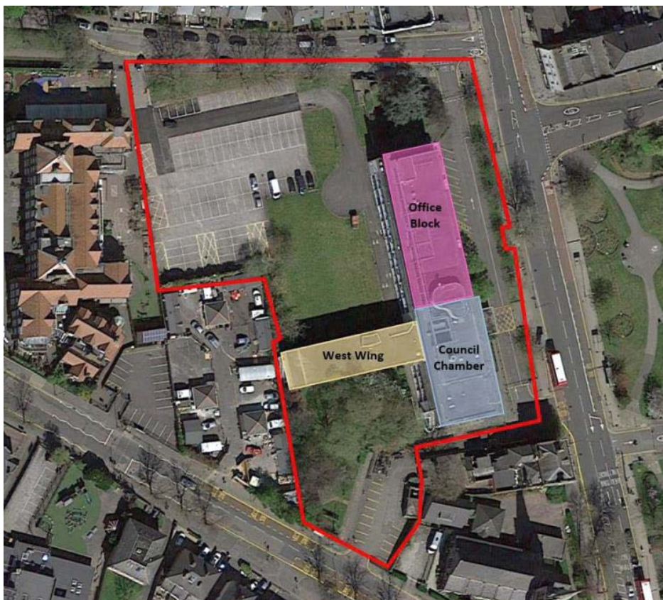
Figure 2-1 Haringey Civic Centre comprising three separate structures (north is up)
