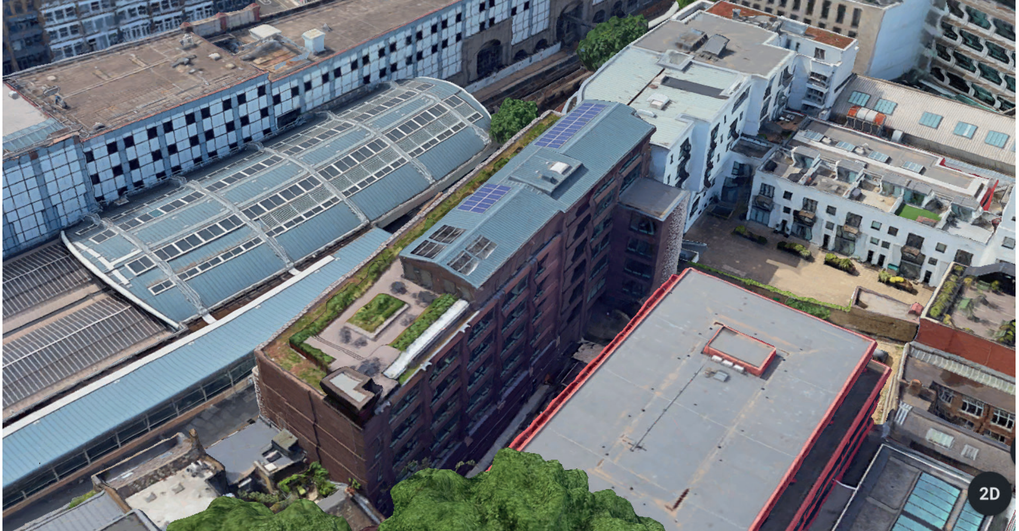
Layden Hosue – Cladding replaced to the front elevation and existing brick walls with internal insulation, on the North, South and west elevation.
