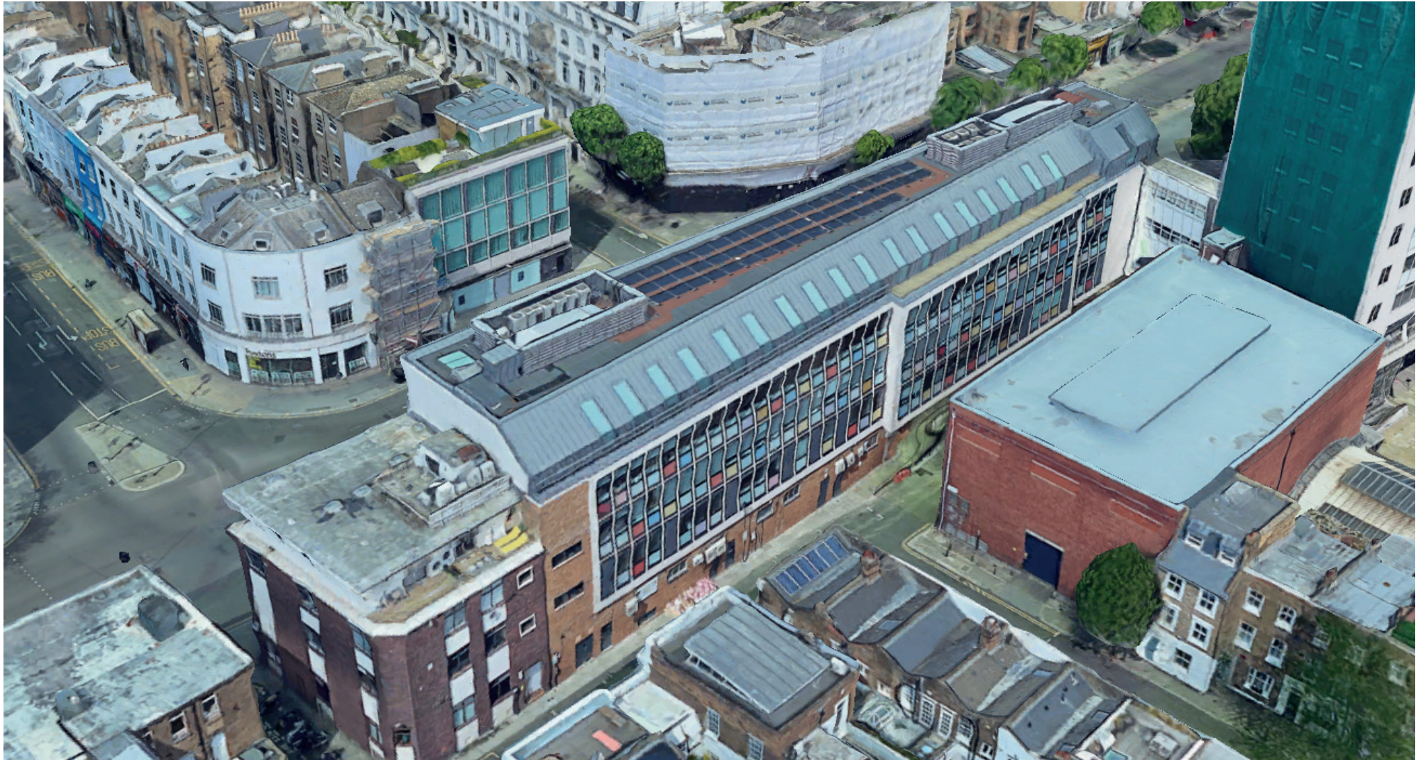
Notting Hill Gate south recladding - west and north wall are retained with internal insulation.
