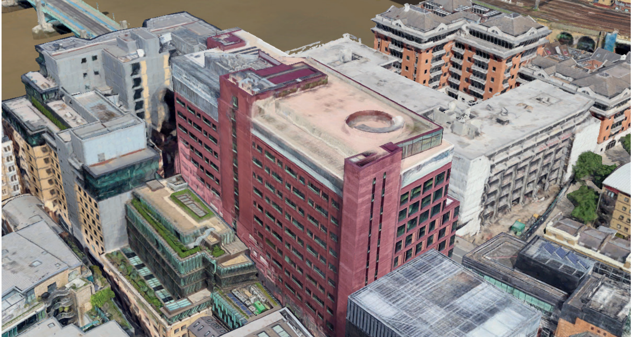
Rose Court – Southwark bridge road. Cladding replaced in the front elevation and brick wall, with internal insulation, on the west elevation.
