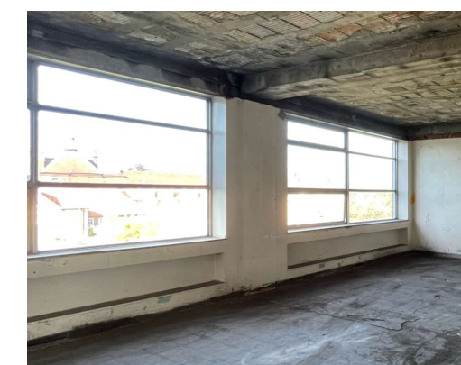
Existing External Wall - L02
