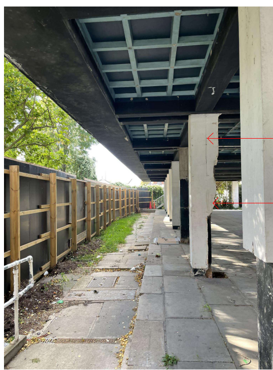
Existing condition below west wing
