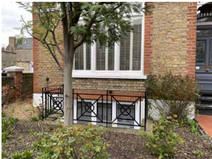
Front light well to 13 Elder Avenue
