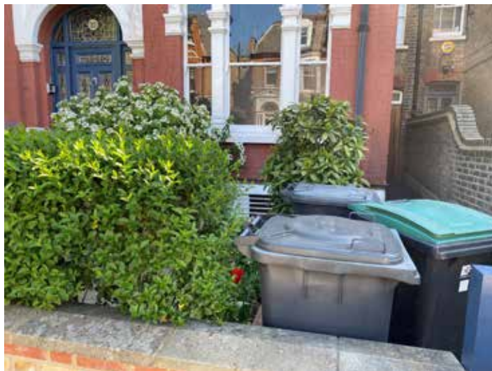
Low level front window / lightwell to 37 Weston Park
