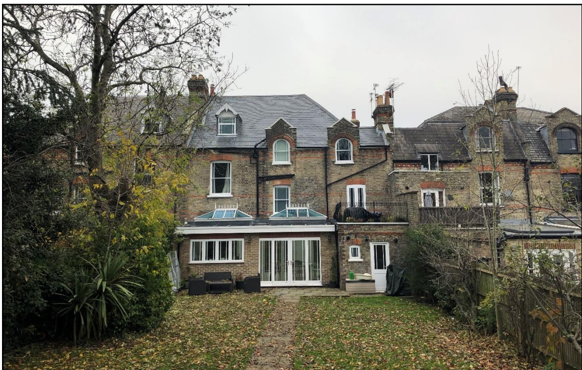
Photograph 2 – Rear view of property
