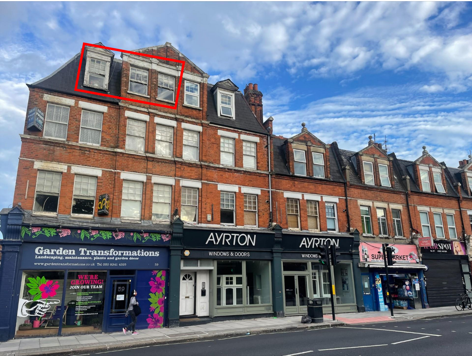
59 TOTTENHAM LANE. FLAT G FRONT VIEW. X3 WINDOWS IN RED BOX
