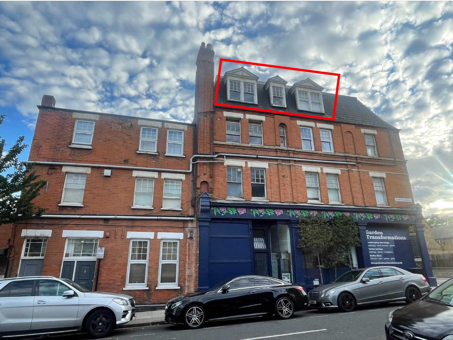
59 TOTTENHAM LANE. FLAT G SIDE VIEW. X5 WINDOWS IN RED BOX
