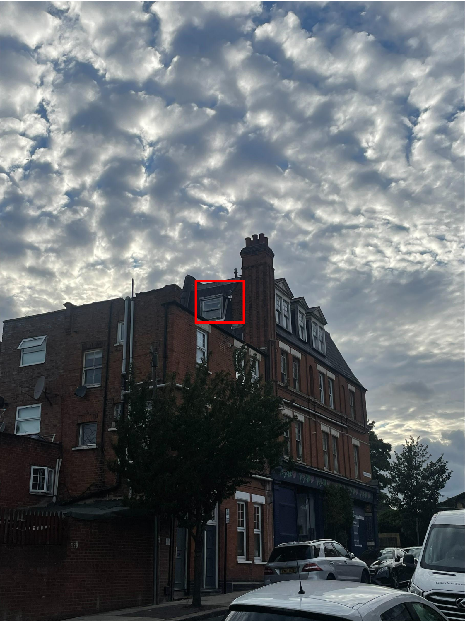
59 TOTTENHAM LANE. FLAT G REAR VIEW. X1 WINDOW IN RED BOX
