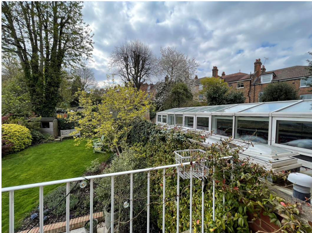
View of the rear / side boundary; view of the nursery roof
