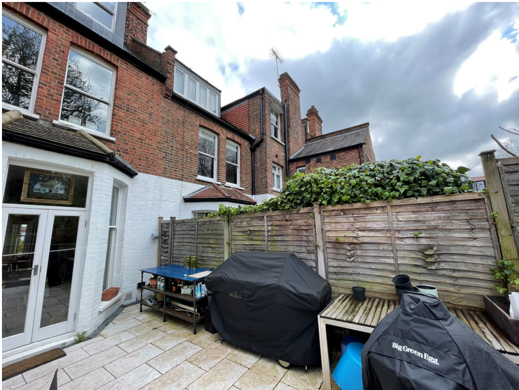
View of the rear / side boundary
