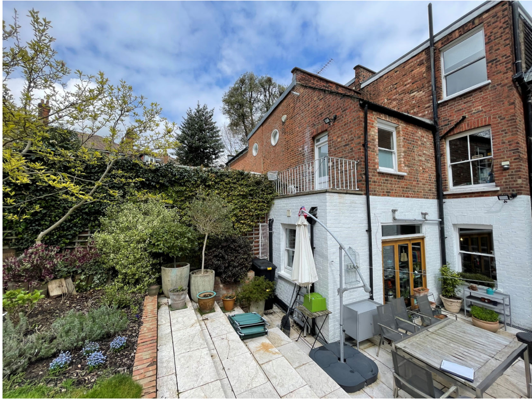
View of the rear / side boundary
