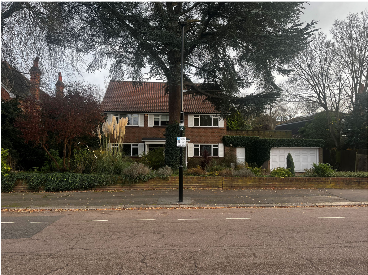
Fig. 1 – Site viewed face on from Stormont Road
