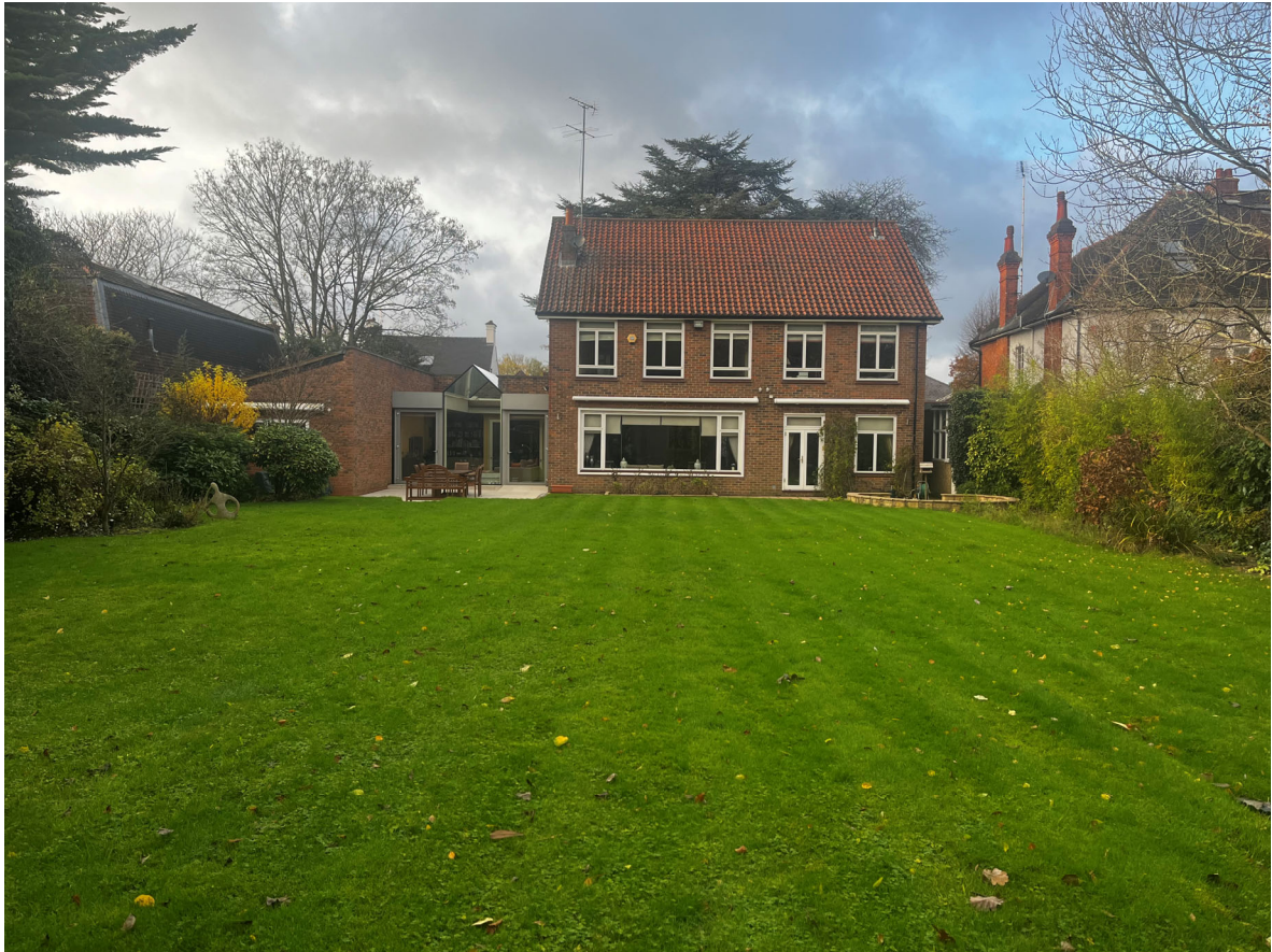
Fig. 2 – House viewed from rear garden
