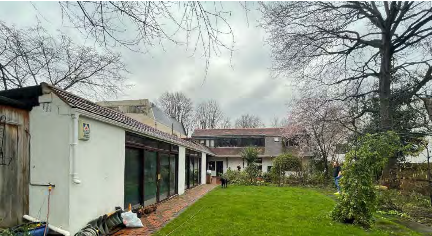
rear extension pool wing.JPG
