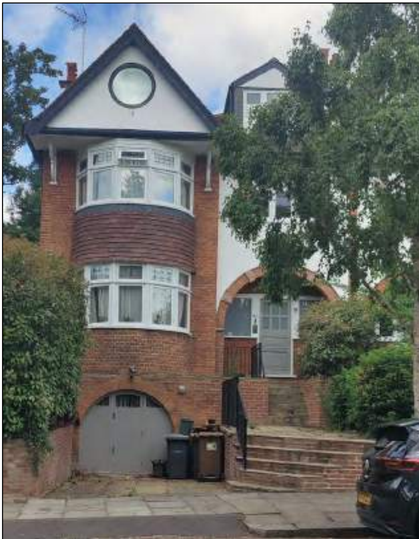
Figure 3.1 Front Elevation (July 2023).
