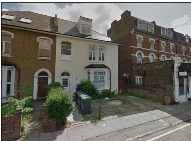
Figure 2: View of property from Alexandra Road
