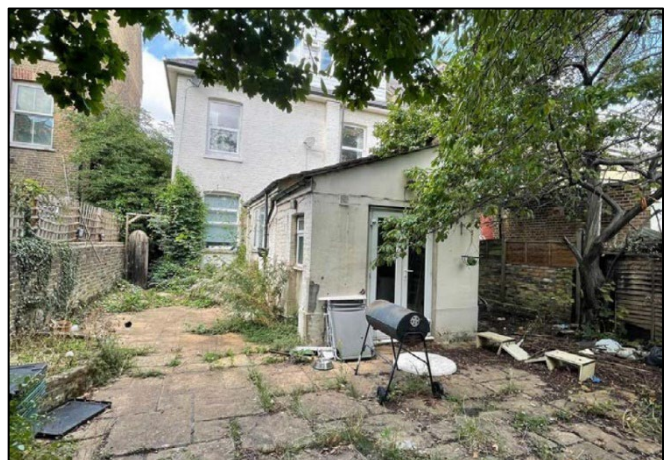
Figure 3: View of rear elevation and extension and rear garden area
