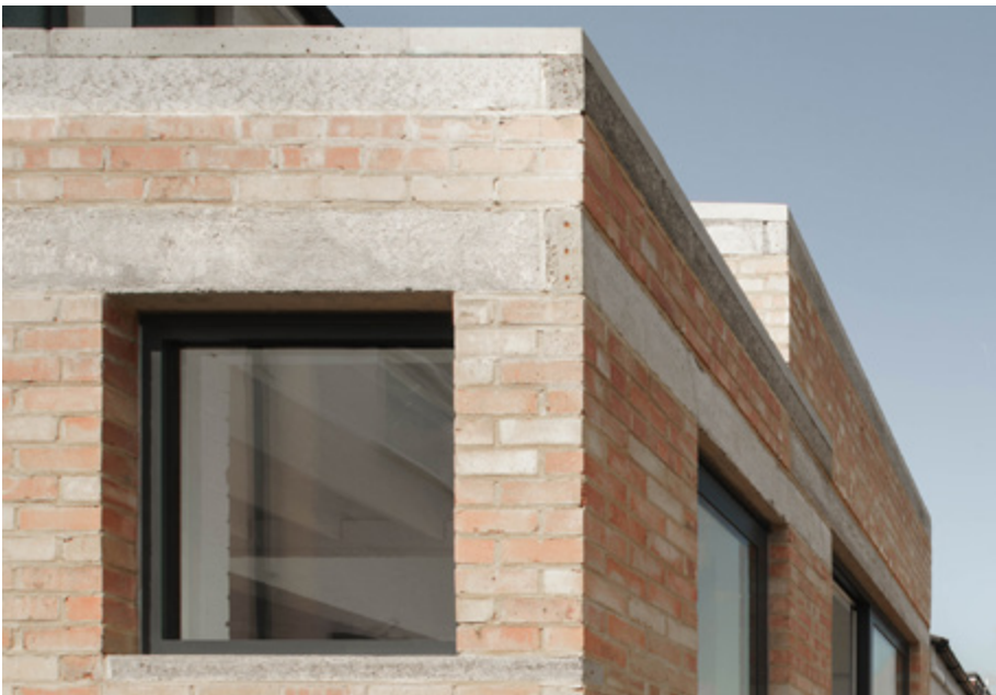
3. Natural concrete finish to cills and lintels
