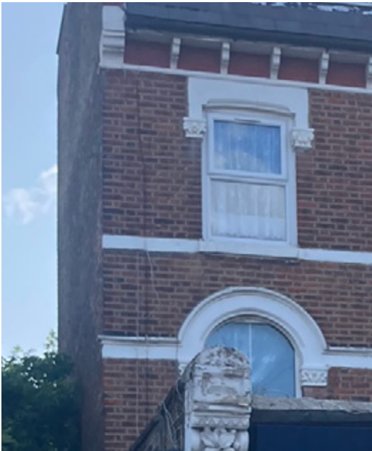
Horizontal white lintels
