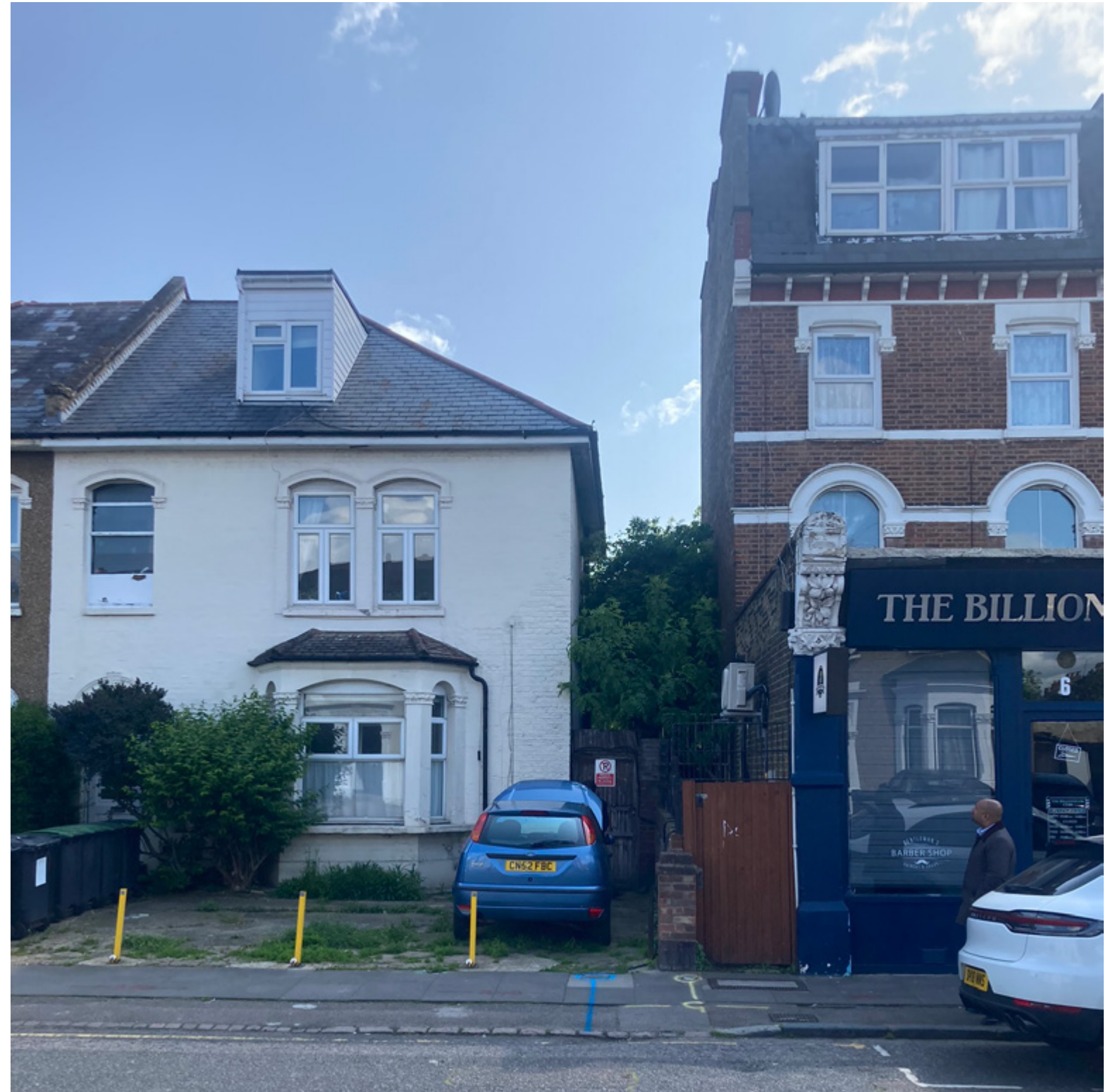
Photo of existing building on 8 Alexandra Road
