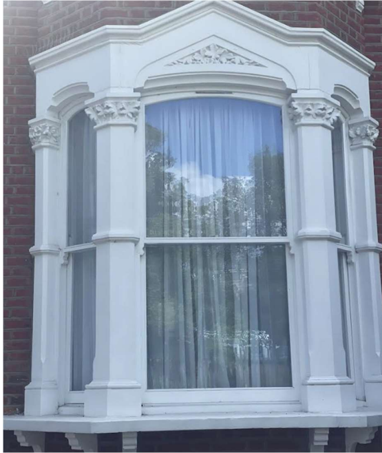
Photograph of existing window to adjoining building
