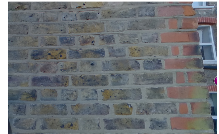
Existing bricks to rear.
