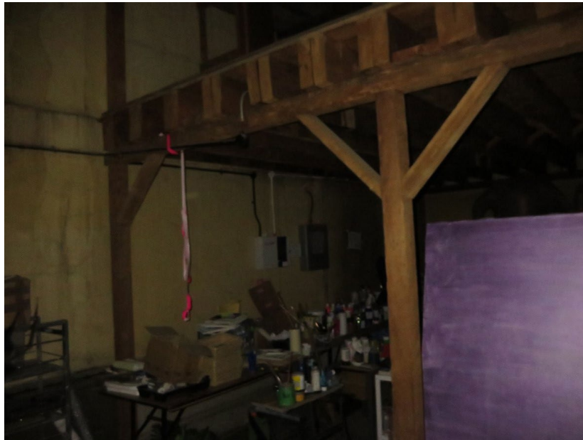
Figure 9: GF SW BBC Store Room (for Changing Places Facility) full height space in front of timber posts supporting mezzanine gantry
