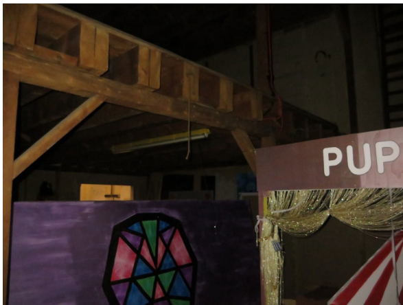
Figure 6: GF SW BBC Store Room (for Changing Places Facility) Looking east toward mezzanine
