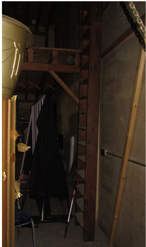
Figure 8: GF SW BBC Store Room (for Changing Places Facility) Looking east toward former ladder access to timber gantry
