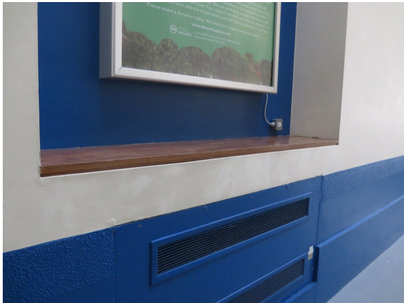
Figure 4: Existing east lightwell
