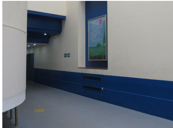
Figure 5: Existing east lightwell
