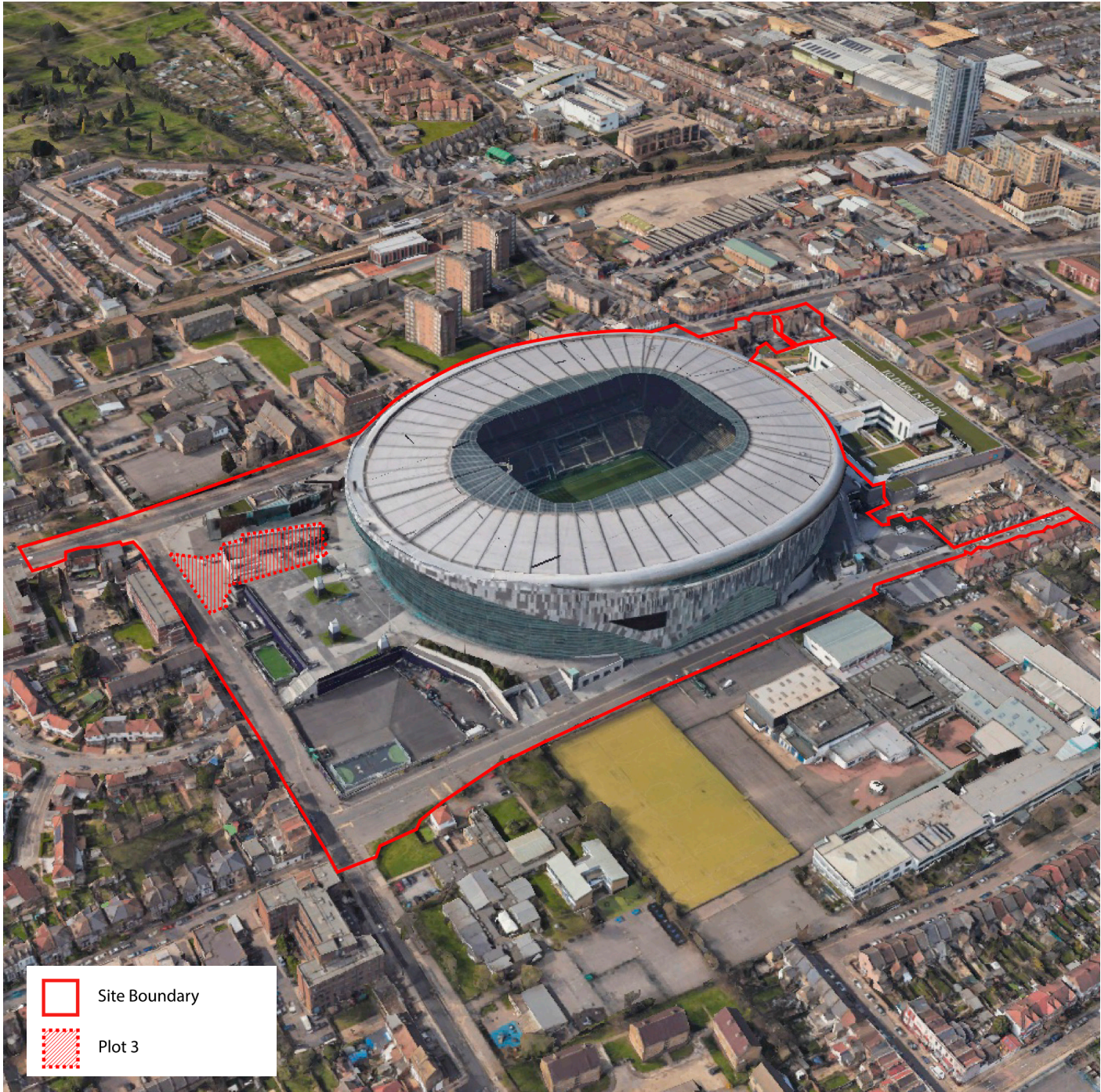
Fig. 3.3: Aerial view of the Site looking northwest (Google Earth, 2023). The Site is outlined in red and the Plot 3 is hatched in red.
