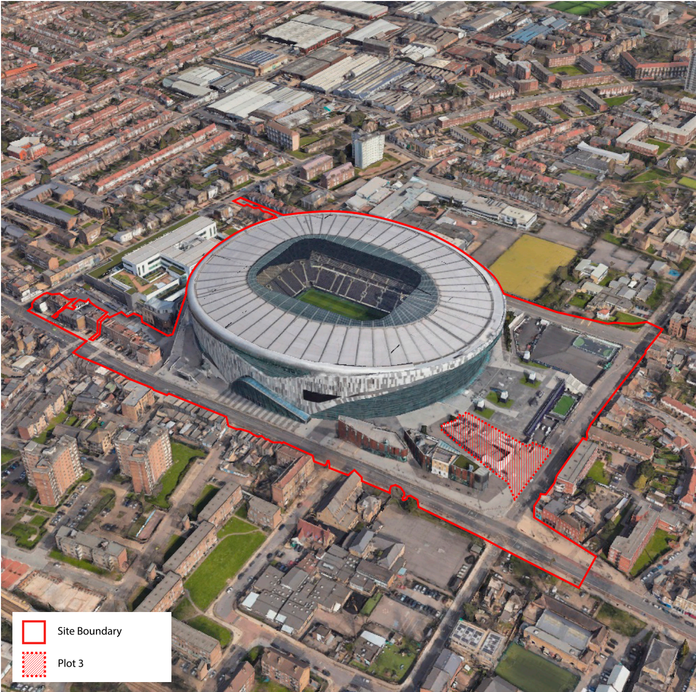
Fig. 3.2: Aerial view of the Site looking north-east (Google Earth, 2023). The Site is outlined in red and the Plot 3 is hatched in red.
