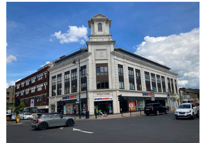
Fig. 6.27: The locally listed building at Nos.636 and 638, the former LCS department store
