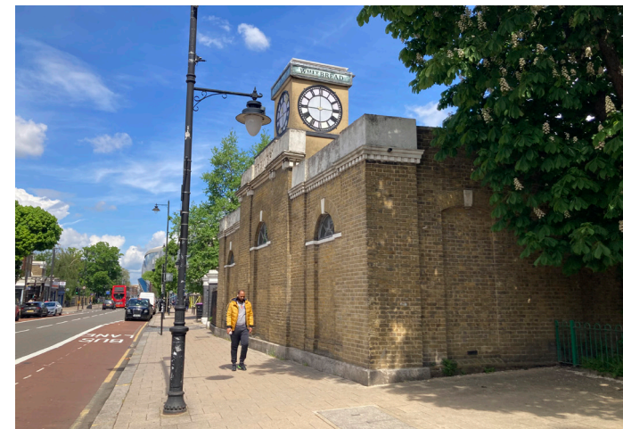
Fig. 6.26: The Grade II listed Southern Gate Building at Whitbread Brewery.
