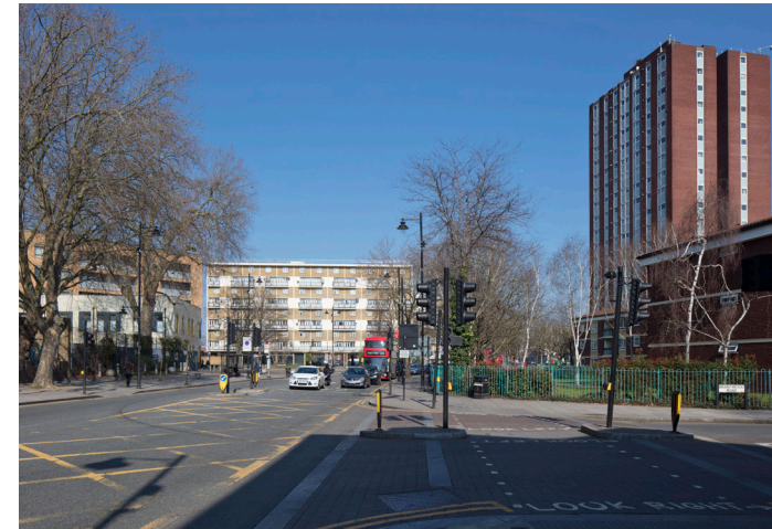
Fig. 6.18: The Brook House Primary School on the left, the Boundary Court building in the centre and the 20-storey Stellar House on the right.
