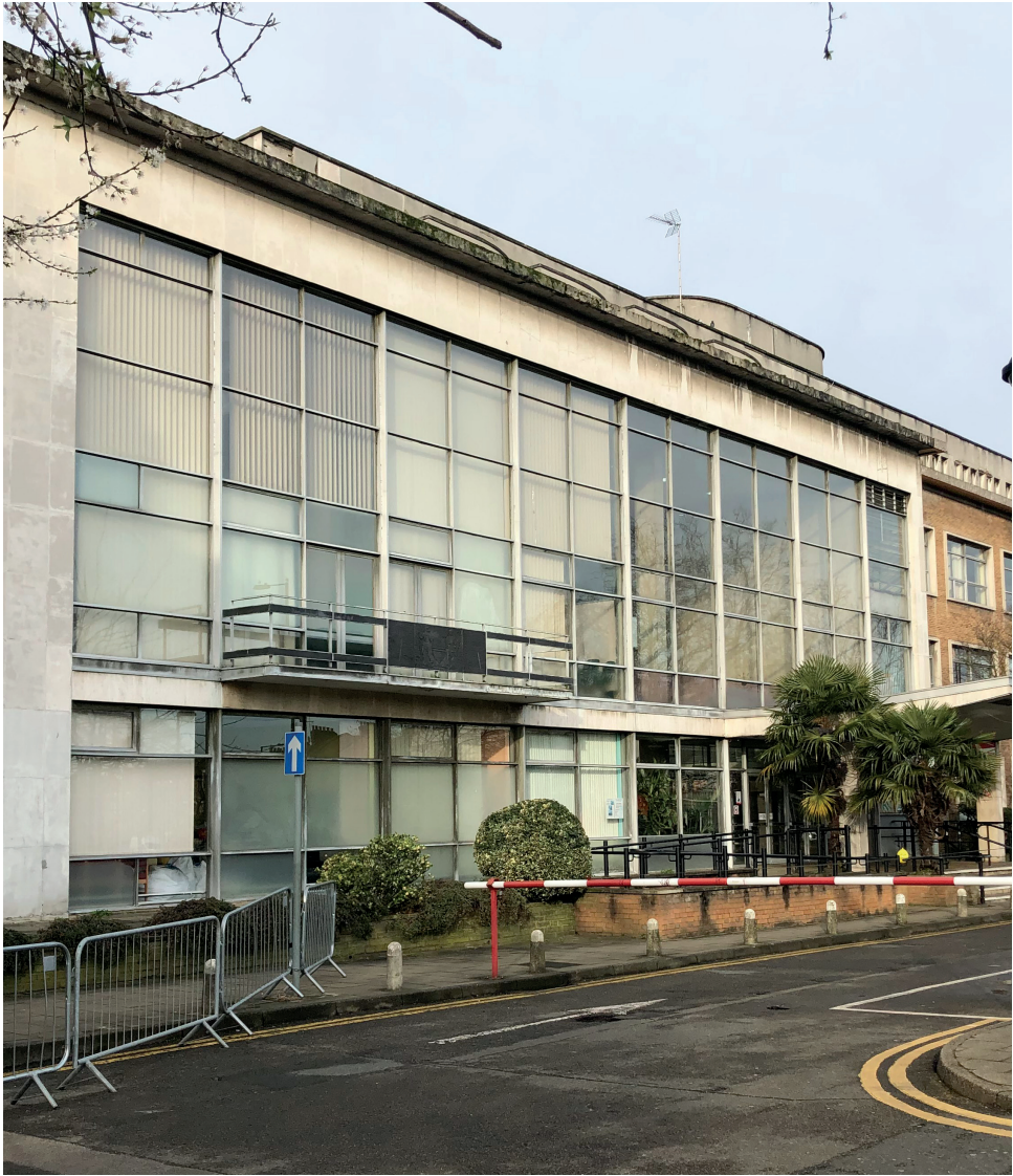
Type 01 Aluminium Curtain Walling System
