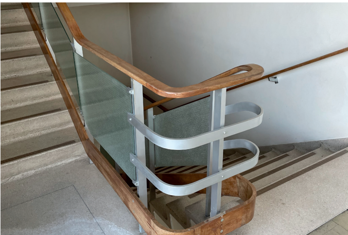
North Stair core
