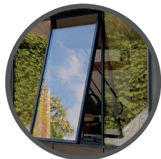
Openable windows for night purge ventilation
