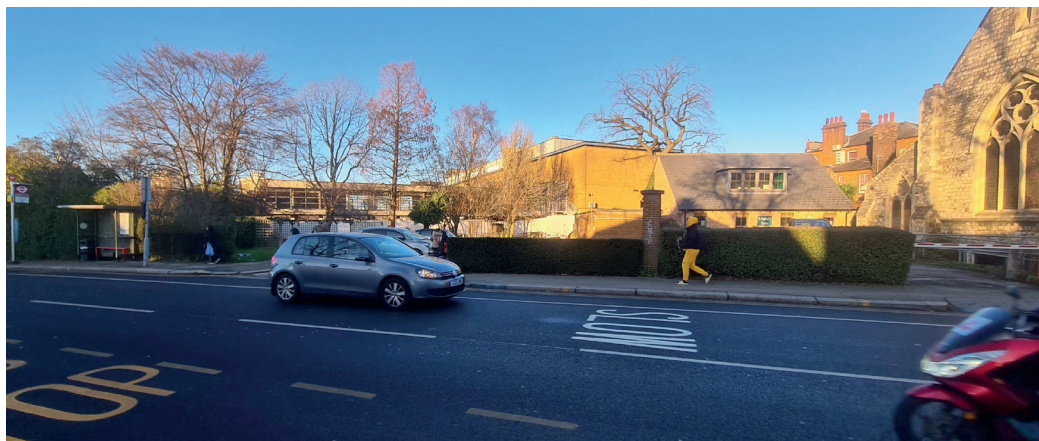
Existing brick wall to rear of Saint Michaels Church extended onto Bounds Green Road frontage
