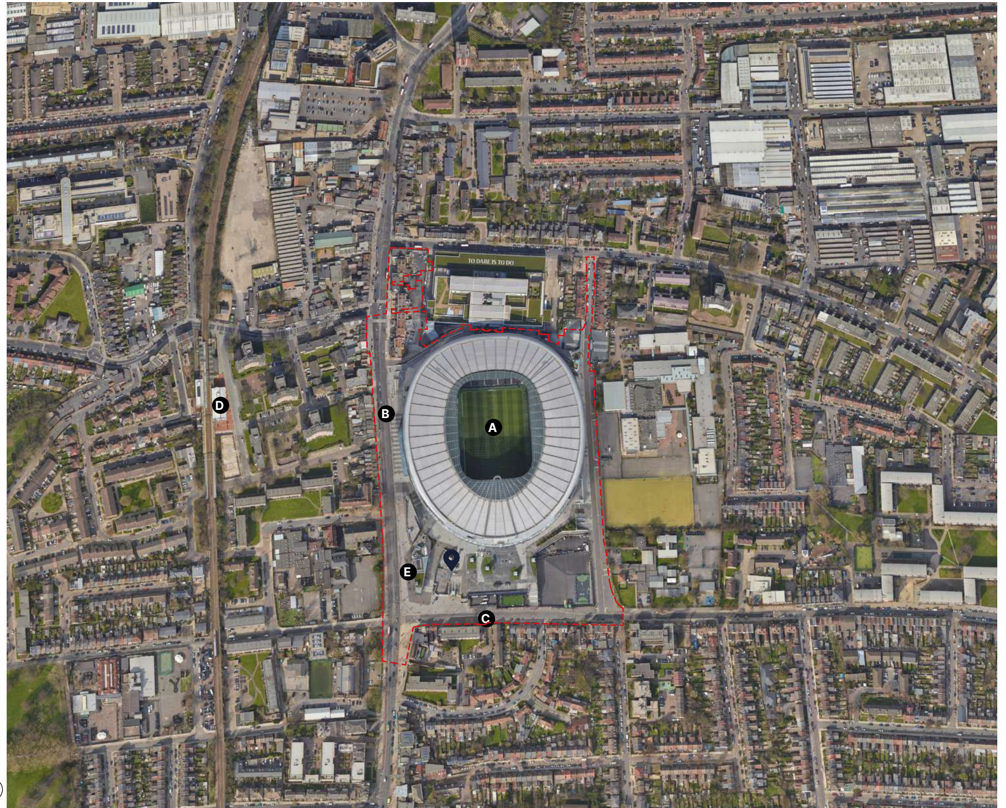
FIGURE 2. Site Aerial Overview
