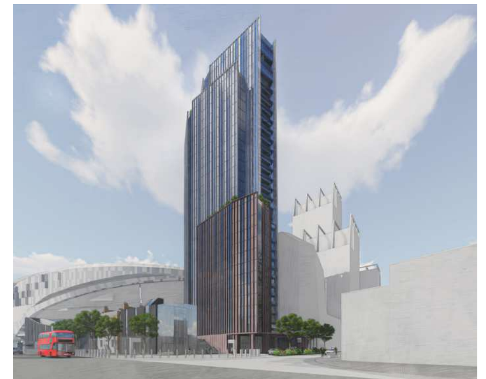
FIGURE 91. View from southern approach
