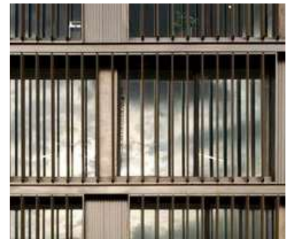
Dark grey coloured Aluminium projected louvres on brise-soleil
