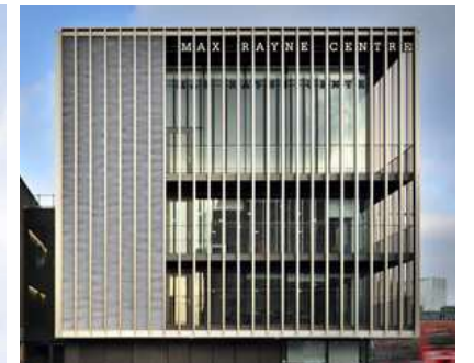
Light Bronze coloured Projected Aluminium Mullions
