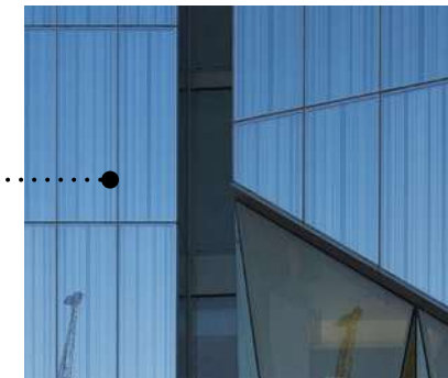
Back-painted and insulated opaque glass colour dark grey
