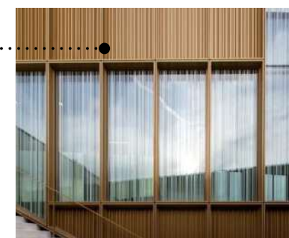
Bronze coloured profiled Aluminium solid panel
