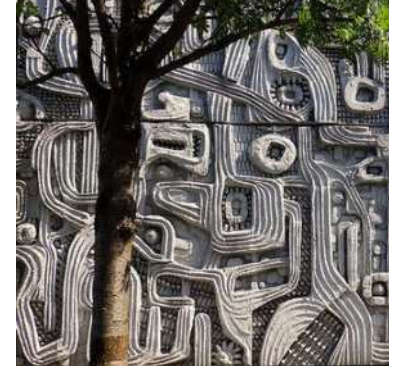
04 Textured Pre-Cast Concrete Panels
