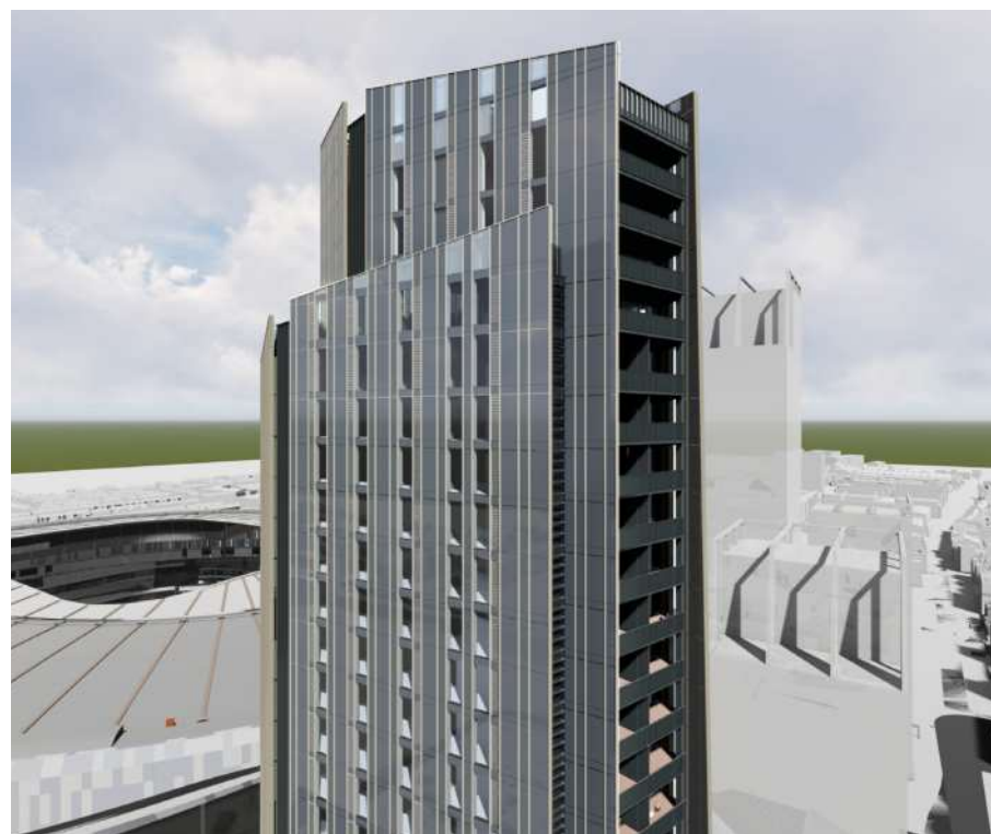
FIGURE 163. Aerial View of Top of Tower
