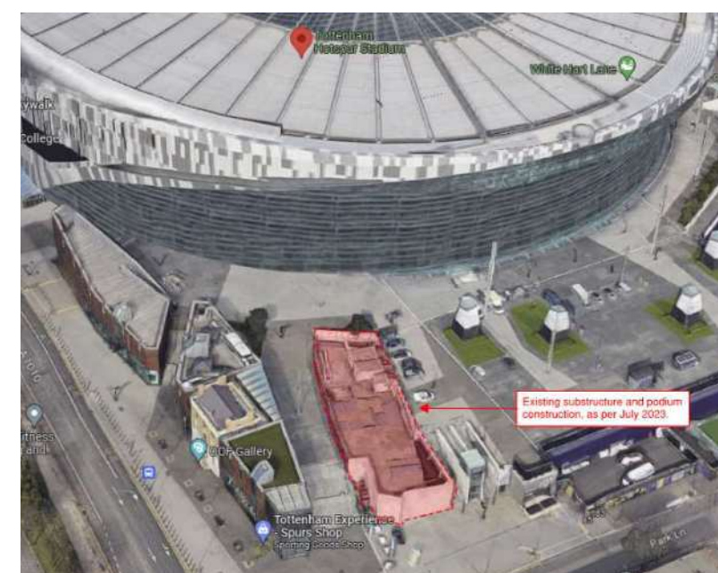
FIGURE 345. Existing structure up to podium Level 1
